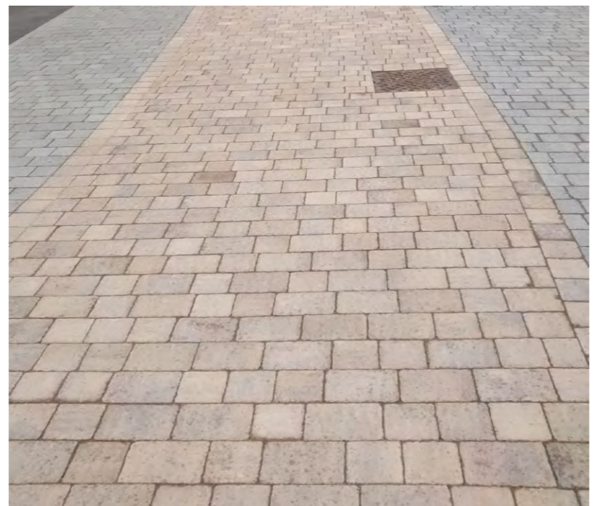
PERMEABLE PAVING TO LOOP ROAD
