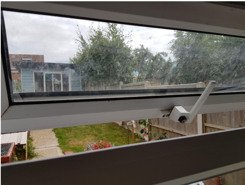
Photo 5: “Open window, hot in summer”. (Loft insulation, Private renter, AW)
