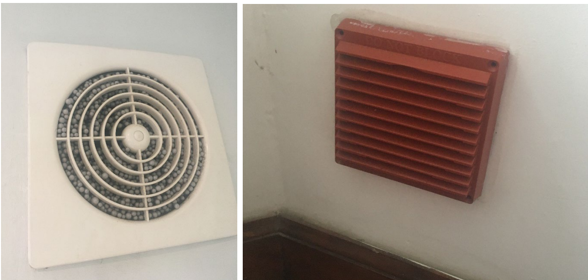
Photo 9: Negative impacts included balls from cavity wall insulation in the kitchen and a vent in the living room causing a draught. (Cavity wall insulation, Owns home, CERO)
