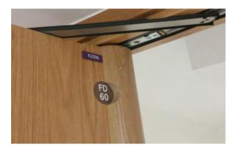
**3: Combined intumescent strip/seal** (image courtesy of Golden Thread Fire Delay)
