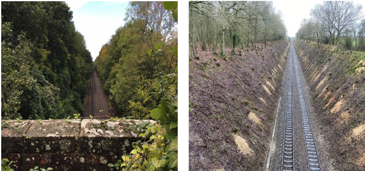
Figure 28: The main lines between Overton and Whitchurch looking towards Salisbury showing the condition of the vegetation before (taken in summer) and after (taken in winter) vegetation work was completed in 2019/20.
