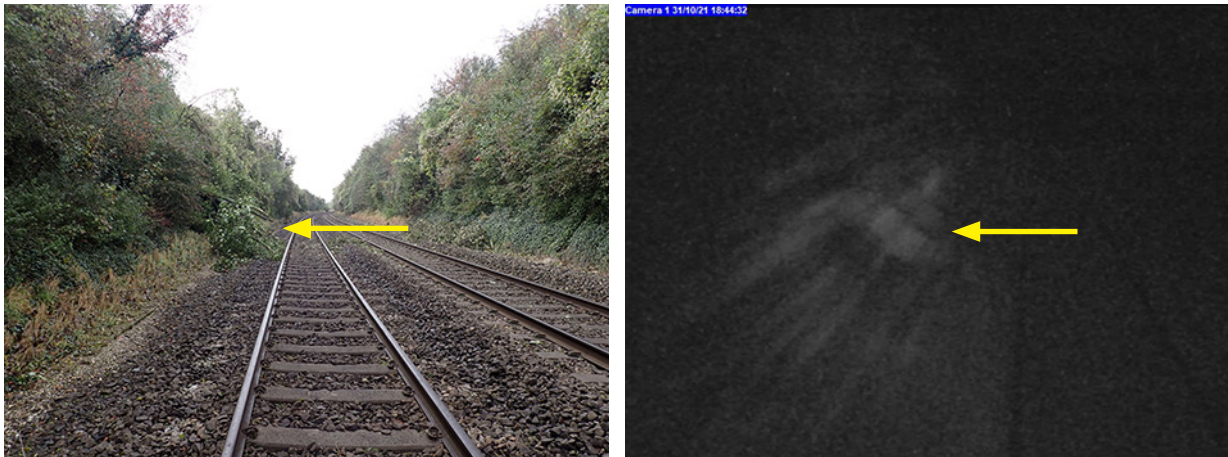
Figure 8: (left) Tree that was struck by train 1L13 (branches had been cut back by the train driver and guard) and later observed by the driver of train 1L53 (when driving train 1L52 on the Up line to London Waterloo) and (right) enhanced image taken from train 1L53 FFCCTV system.
