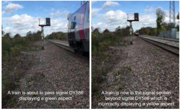
Figure 11: Stills from the video footage recorded by the local signalling maintenance team showing signal DY586 displaying the incorrect aspect (courtesy of Network Rail).
