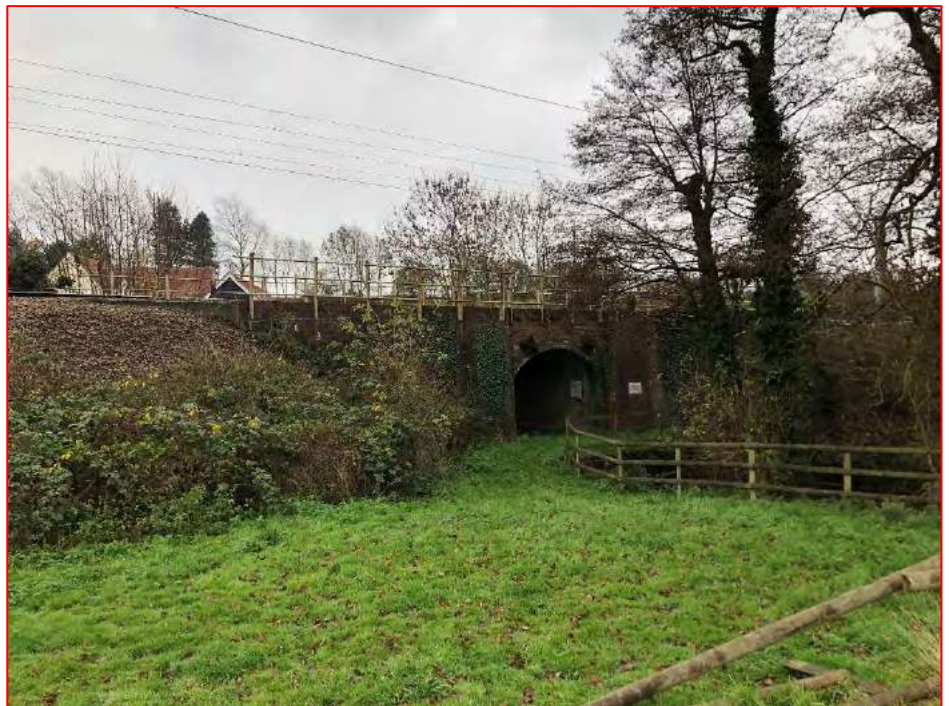
Plate 11 Looking southwest towards railway bridge
