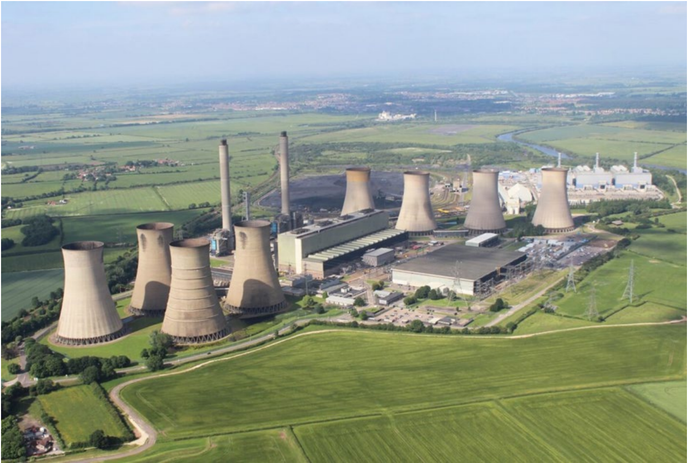
Figure 13 – The West Burton site before being developed for STEP
