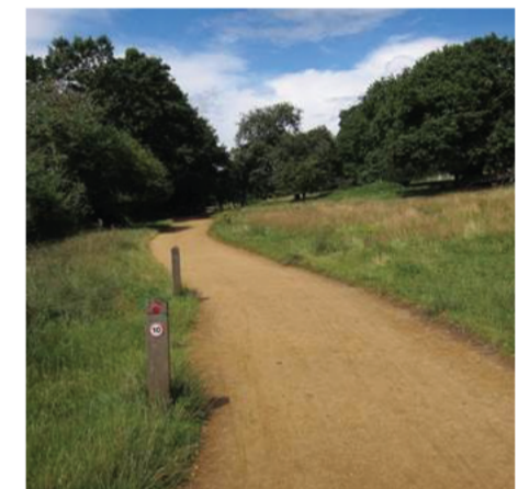
Figure 1. Typical loose aggregate footpath, buff colour. Timber bollards to be positioned at regular intervals adjacent to cycle paths to denote max speeds.
