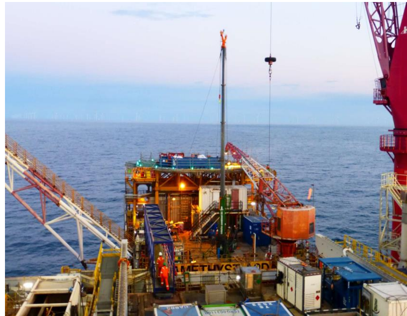
Figure 1: Decommissioning activity at Amethyst A2D
