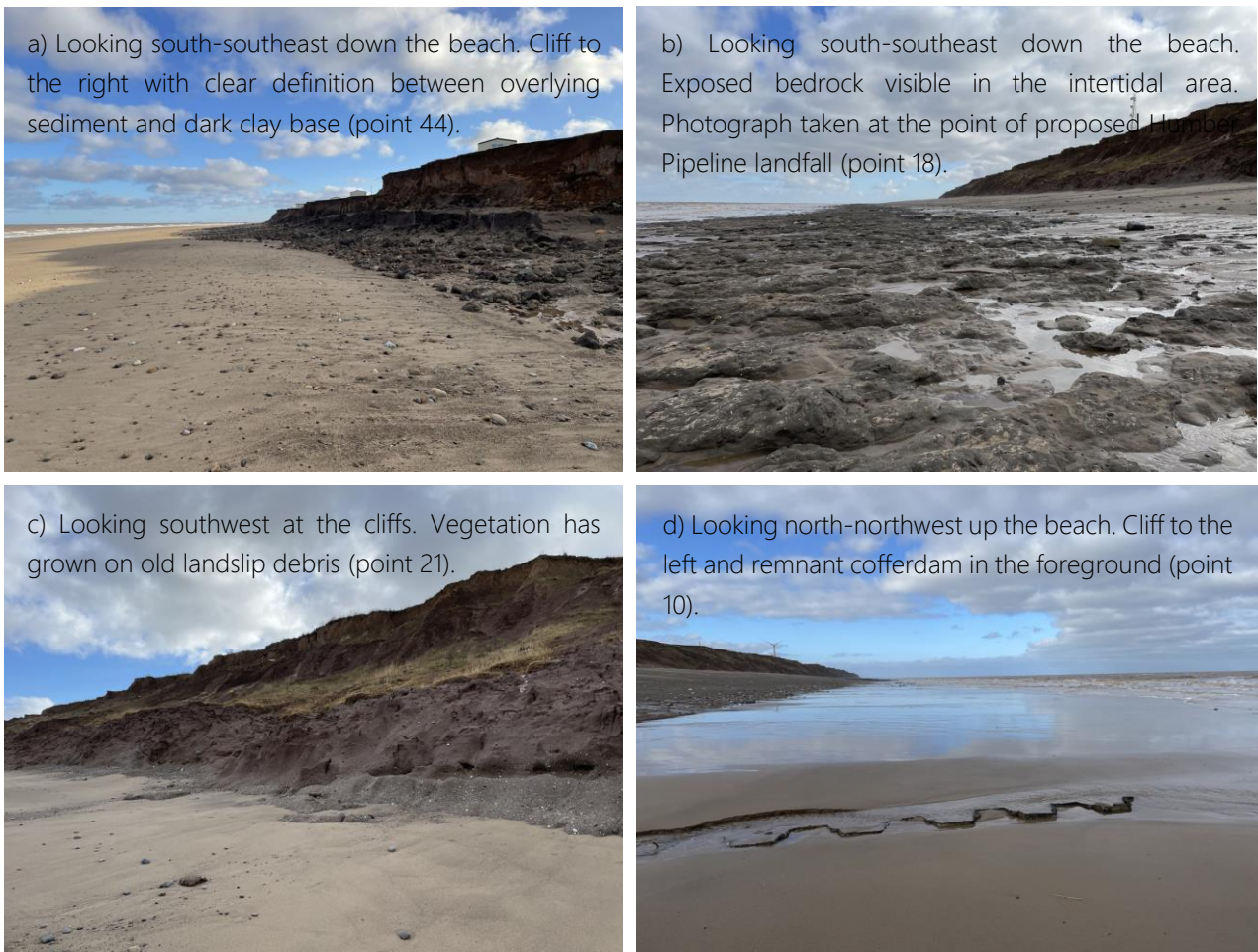
Figure 2-31 - Humber site visit photos (point numbers are shown on Figure 2-29)
