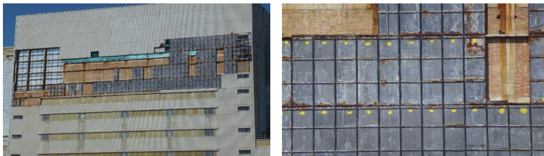
Reactor 2 south face following phase 1 repairs to make the buildings
