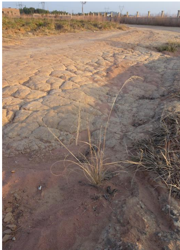
Figure 47 – Detail of soil erosion in Ferrasols along an access road (eastern region).
