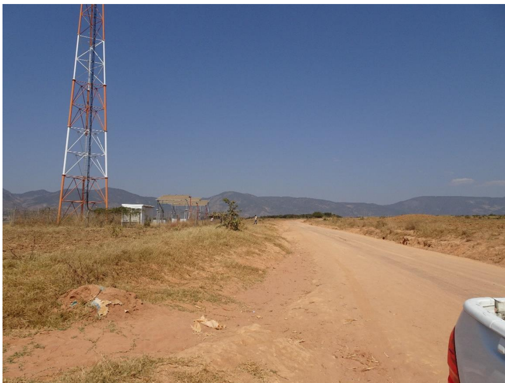
Figure 49 – Unpaved road in the project corridor.
