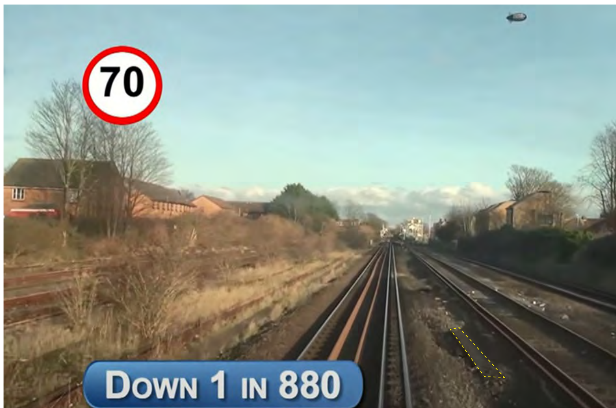
Figure 9: Still image of the detached conductor rail board taken from a video uploaded to YouTube 27/10/2016 (courtesy of Paul Hubbard).
