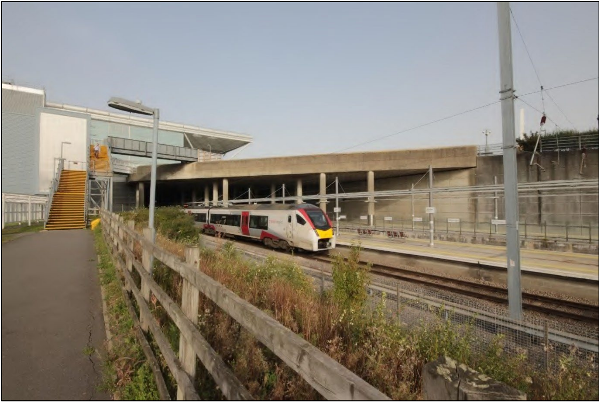
Photograph 3: View of the train lines running under the Stansted Terminal building, taken facing east
