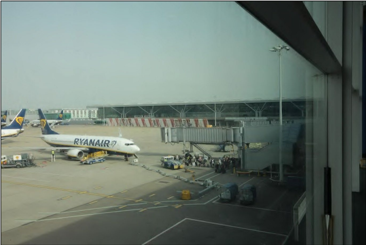
Photograph 25: View towards the Terminal's northwestern elevation from Satellite 2, taken facing east
