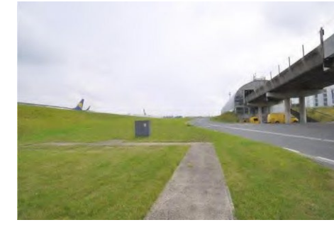
Existing Track Transit System Maintenance Building
