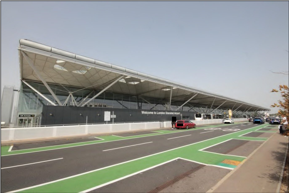
Photograph 17: Oblique view of the south-east elevation of the Terminal, taken facing north
