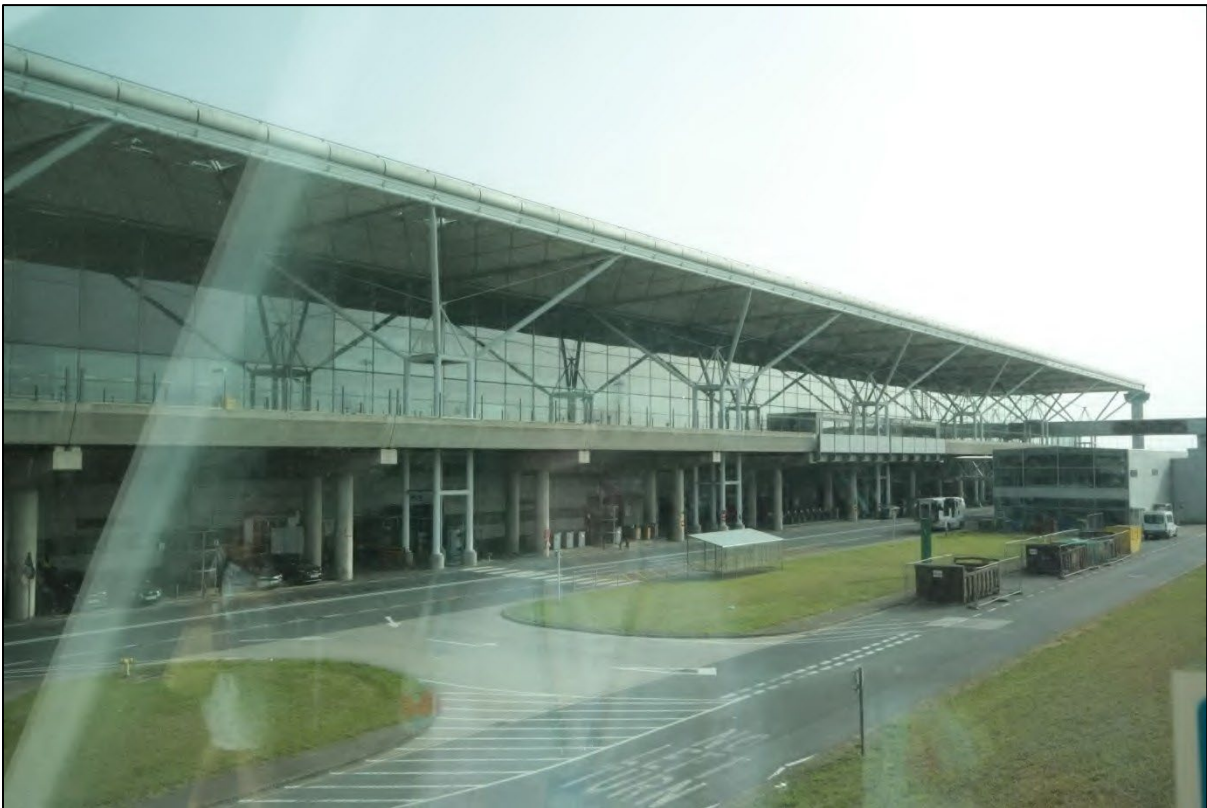
Photograph 24: Oblique view of the Terminal's northwestern elevation, taken facing south from the sky link to Satellite 3
