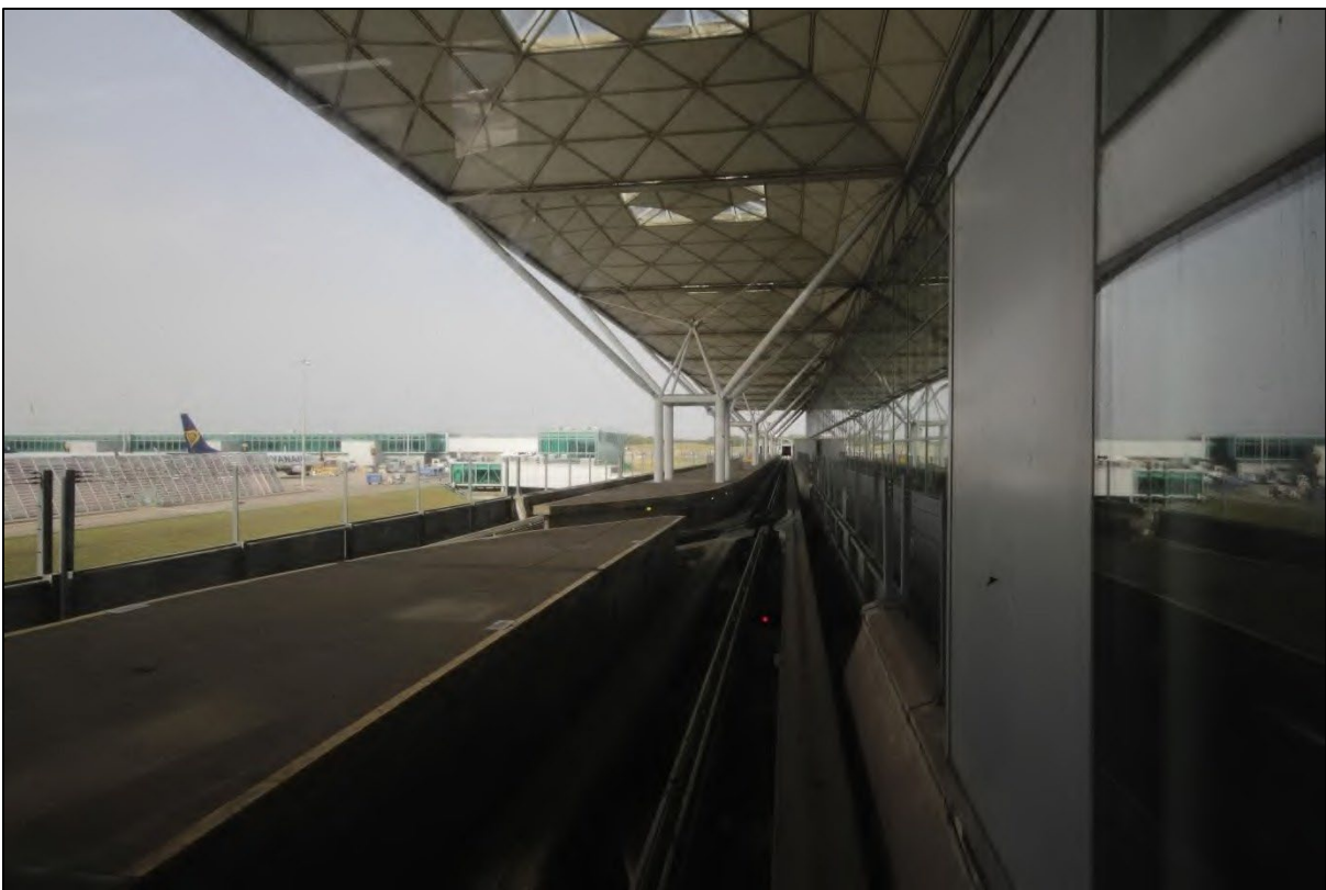
Photograph 16: View of the overhanging canopy to the north-western side of the building, taken facing northeast
