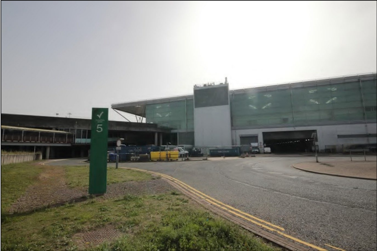
Photograph 23: View of the southern extent of the Terminal building's northeastern elevation, taken facing south
