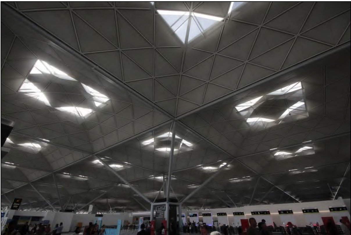
Photograph 10: View of the modular roofing within the building, taken facing west
