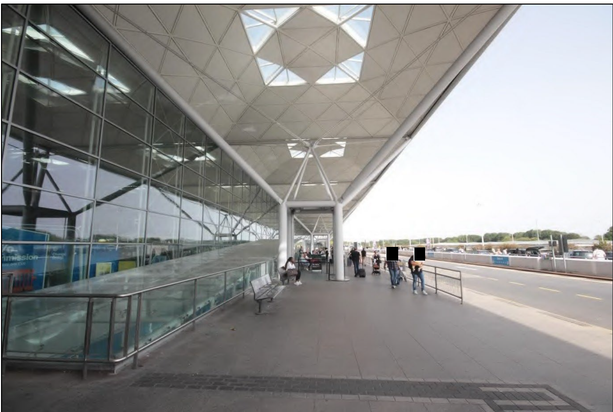
Photograph 20: View beneath the canopy of the Terminal building's south-eastern elevation, with the glazed structure sloping down to the train station
