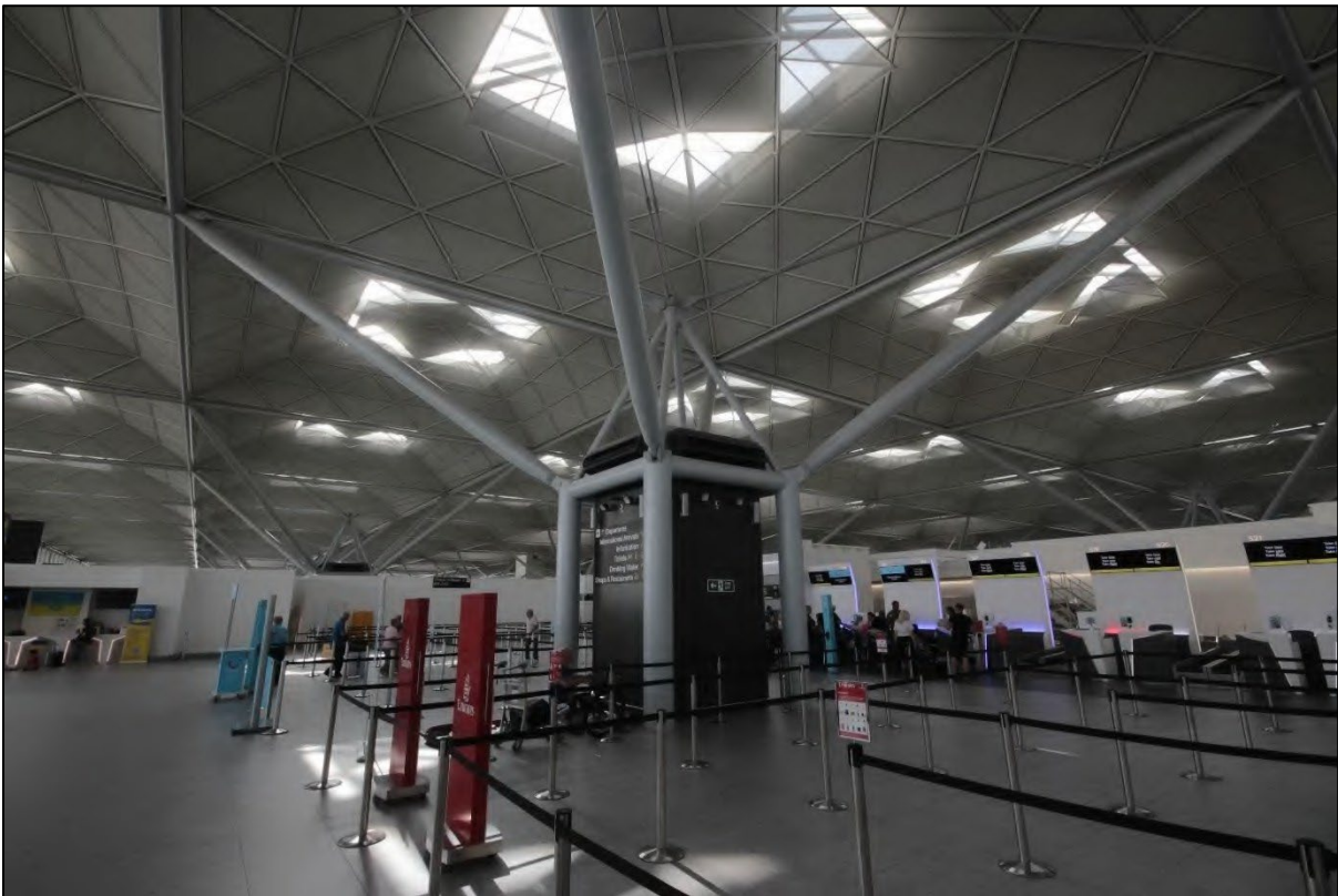
Photograph 12: View of one of the structural steel 'trees' within the Terminal building, taken facing west
