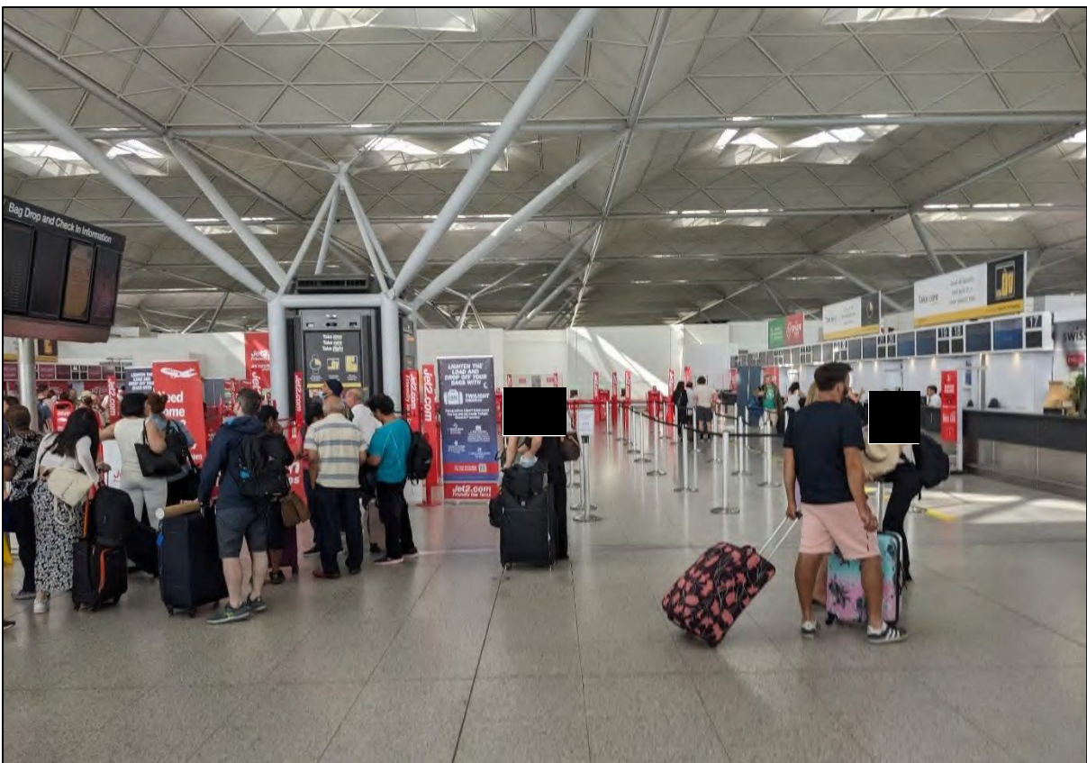
Photograph 32: View to the northwest at concourse level, showing the lack of visibility to the other side of the building
