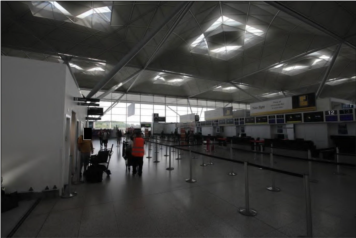
Photograph 29: View to the south at concourse level
