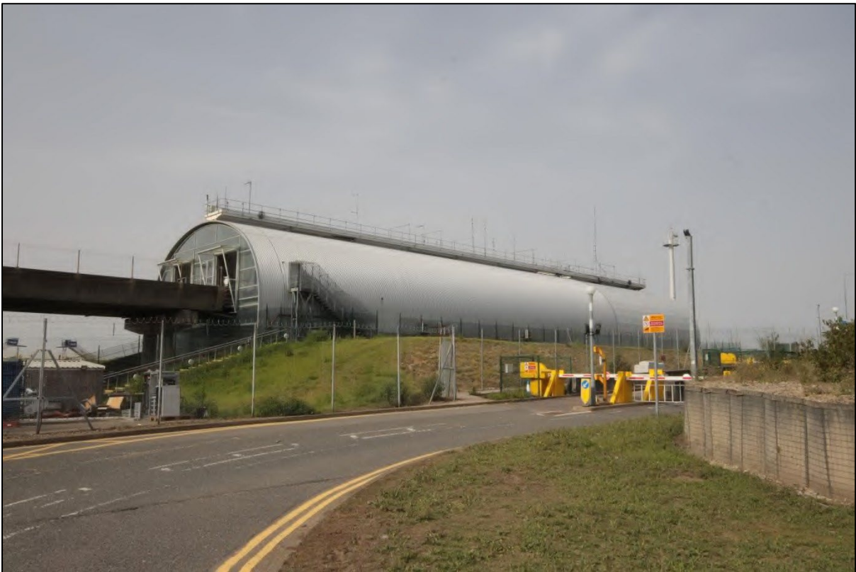
Photograph 7: View of the maintenance building to the north-east of the Terminal, associated with the TTS system
