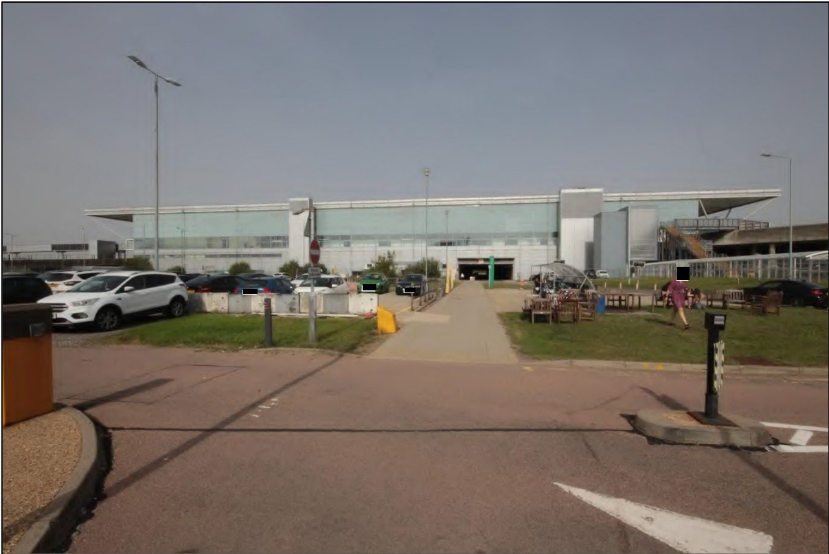
Photograph 27: View of the southwestern elevation of the Terminal building, taken facing northeast
