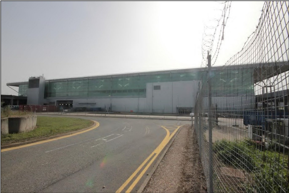
Photograph 21: Oblique view of the Terminal building's northeastern elevation, taken facing south
