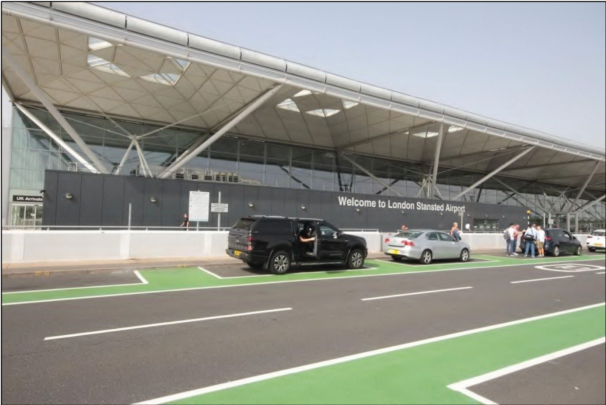
Photograph 19: View towards the single-storey temporary building attached to the western extent of the south-eastern elevation. Taken facing north
