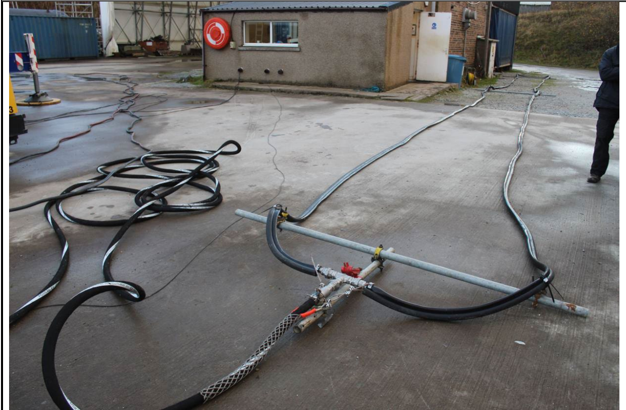
Figure 2-6 Bubble curtain assembly
