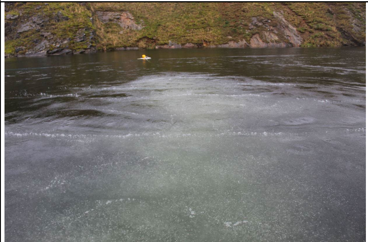
Figure 2-8 Bubble curtain with air compressor at fully output – close up
