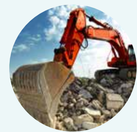
Final stages of decommissioning and clean-up
