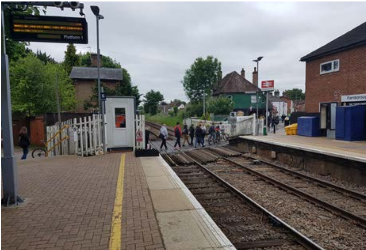
Figure 6: View looking south along platform 1 (not on the day of the incident) showing passenger information screen, crossing attendant's cabin and footpath crossing.
