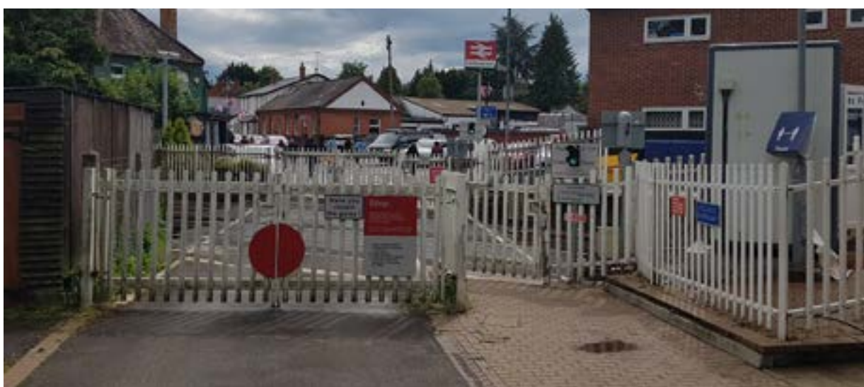
Figure 4: View looking west from near platform 1 showing user worked crossing (left), footpath crossing (centre) and side of crossing attendant's cabin (right).
