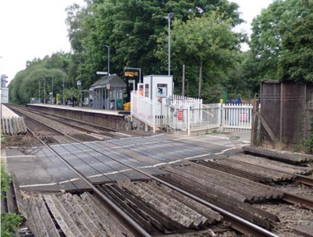
Figure 12: Crossing keeper's cabin within a fenced compound.
