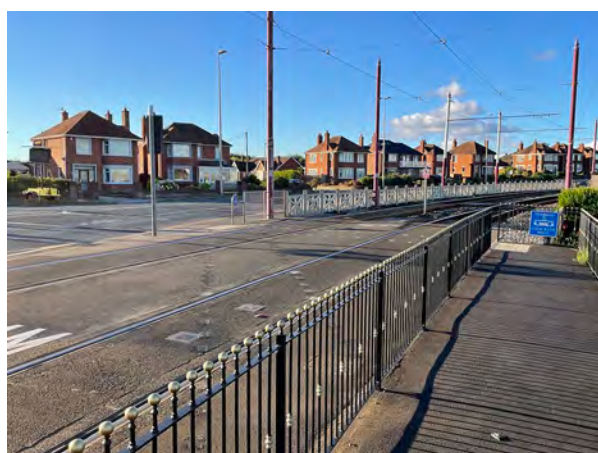
Figure 9a: The revised crossing layout, photographed from the western end of the previous crossing, with remains of previous crossing markings visible.
