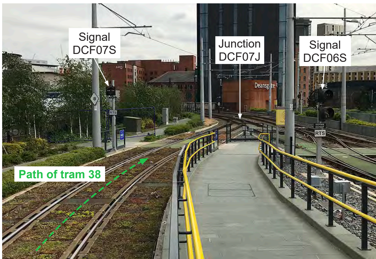
Figure 5: Signal DCF07S located beyond the inbound platform
