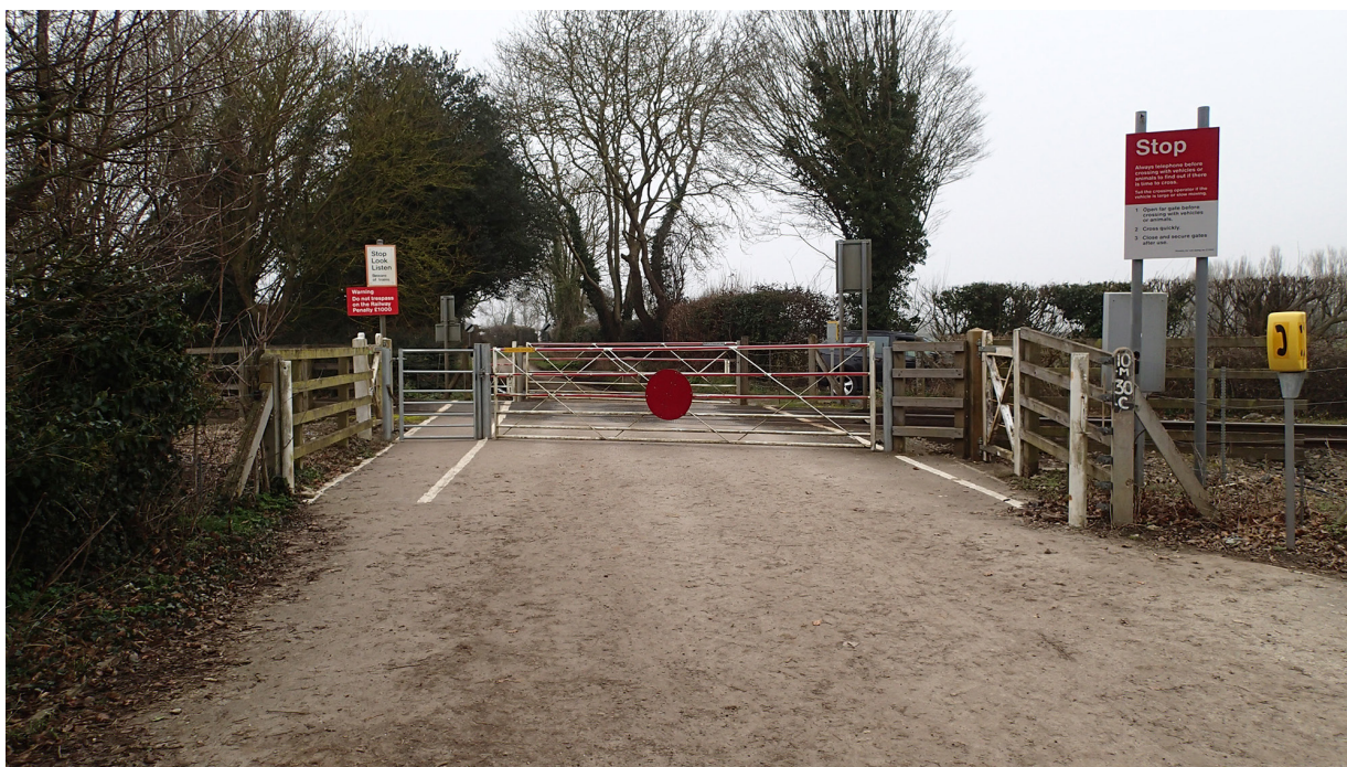
Figure 3: Coltishall Lane user worked crossing viewed from the east, in daylight with closed gates
