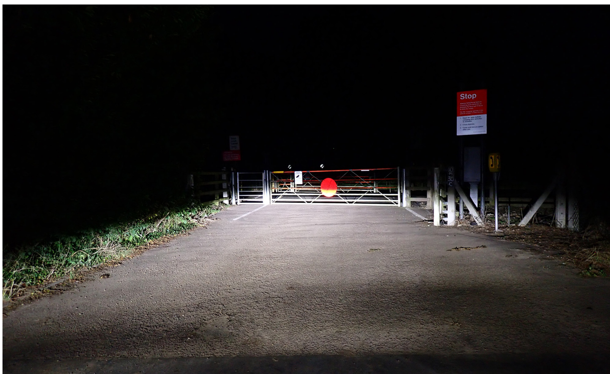
Figure 7: The view of the east side of the crossing from 10 metres away in darkness with gates closed. (The white sign on the gate has been added since the date of the incident)
