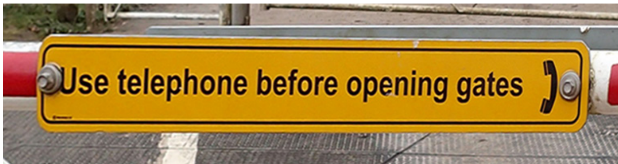
Figure 9: The additional sign added to the road gates close to the latch
