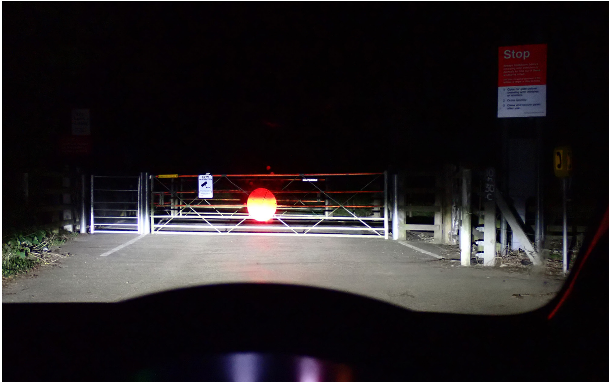
Figure 8: The view of the east side of the crossing from 5 metres away in darkness with gates closed. (The white sign on the gate has been added since the date of the incident)
