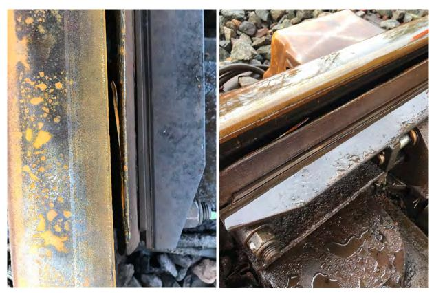
Figure 17: Damage to the switch tip of points 997A
