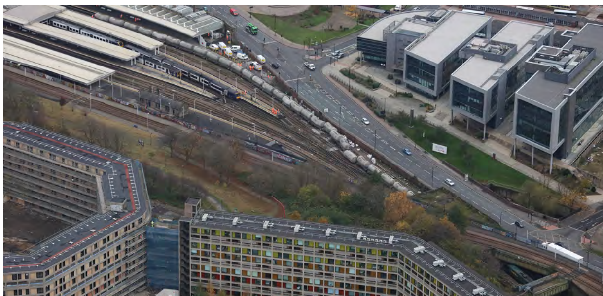
Figure 2: Aerial overview of the derailed train (image courtesy of Network Rail Air Operations team)
