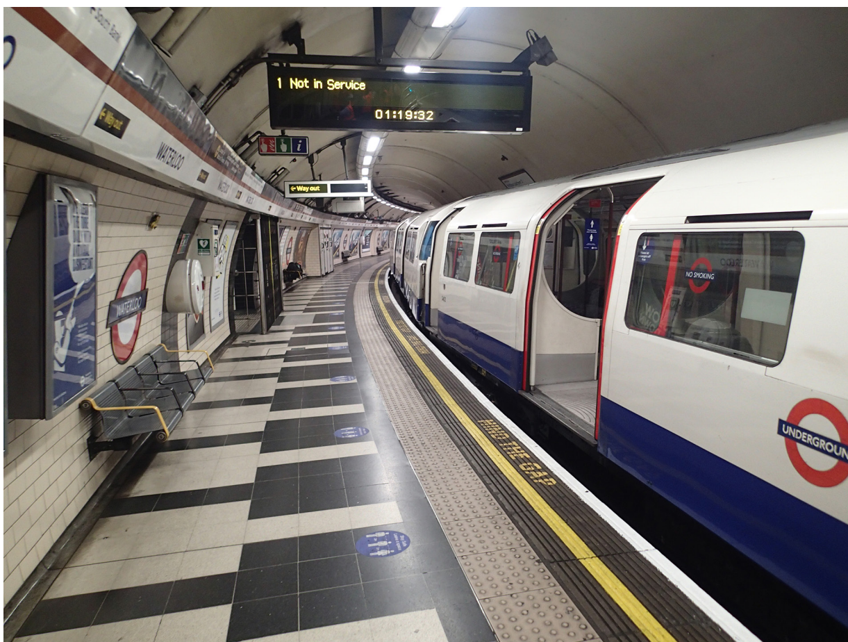
Figure 3: View of Waterloo Bakerloo platform 3 looking south showing the platform curvature and gap between platform and vehicle body
