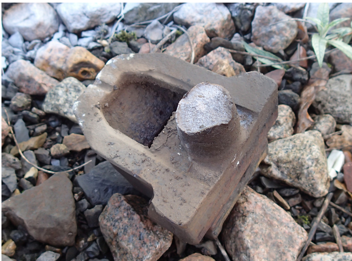
Figure 8: Photograph of one of the failed cast iron shoulders
