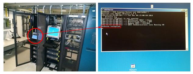
Figure C5: Computer terminal located within the GEST server equipment enclosure at Machynlleth control centre (left image) and unknown exception message seen on laboratory system (right image)
