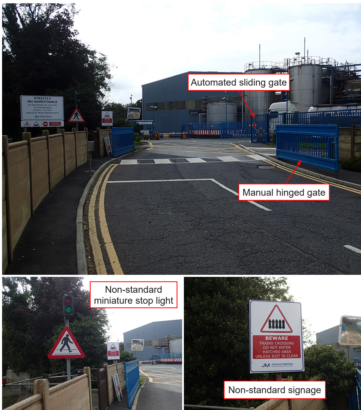
Figure 17: The non-standard features at the Johnson Matthey level crossing
