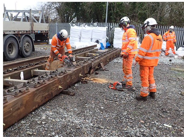
Figure 17: Timber 2L being cut into sections for examination
