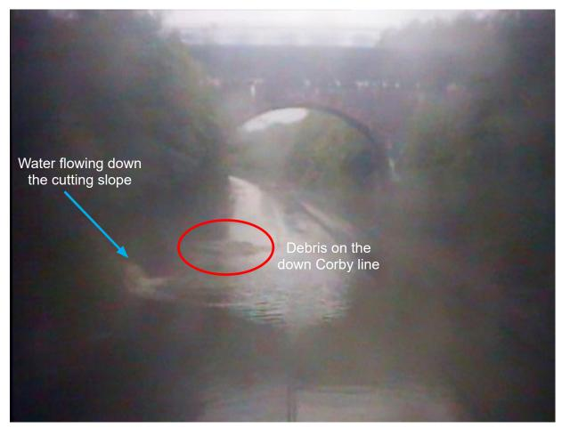
Figure 7: Image from the forward facing CCTV on train 1D43 showing the flooding and debris on the down line.
