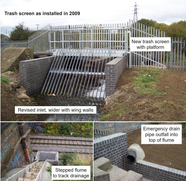
Figure 18: The changes made at the aqueduct's entrance, 2007-2009 (images courtesy of Network Rail)
