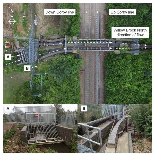
Figure 4: The aqueduct over the railway
