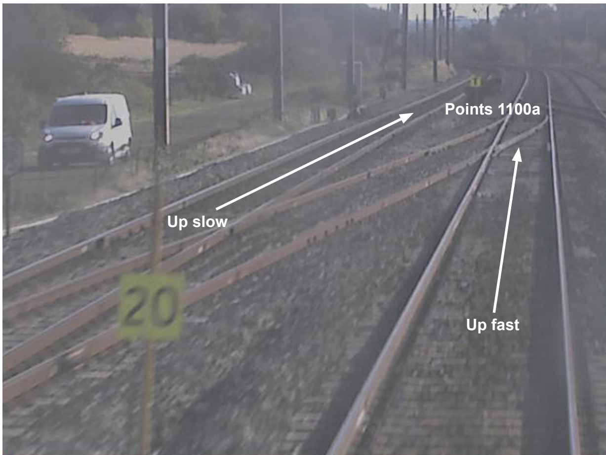
Figure 2: Forward facing closed-circuit television view of points 1100A and its associated crossing on the East Coast Main Line at Sandy South Junction annotated to show key features (image courtesy of LNER)
