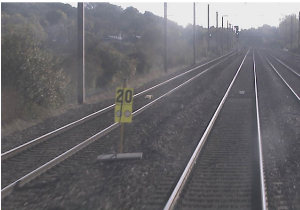
Figure 9: FFCCTV view of the warning board (image courtesy of LNER)
