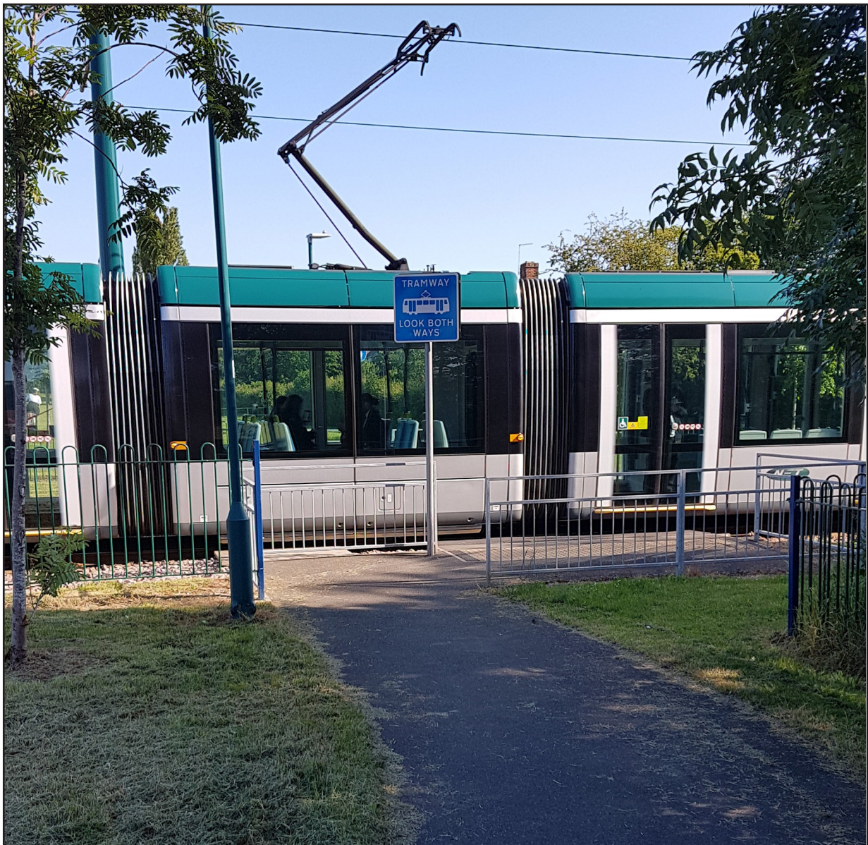
Figure 12: An example of chicane fencing on a footpath crossing on the Nottingham tram system. The tram in the picture is travelling on the closer of the two tracks from right to left.
