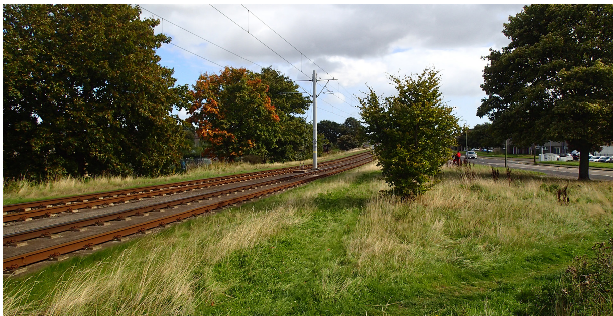
Figure 6: The view to the east from the footpath at 6 metres from the crossing
