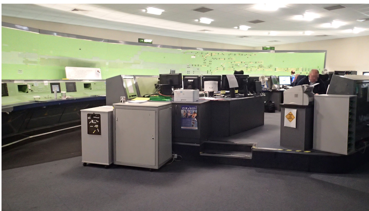
Figure 9: London Bridge signal box operating floor
