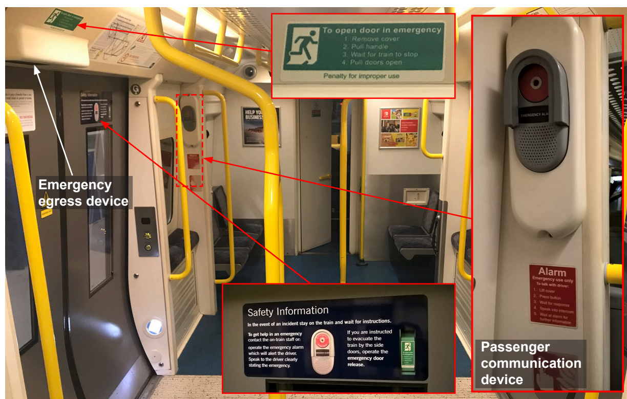
Figure 15: Passenger vestibule on class 376 unit (images courtesy of London and South East Railway Ltd)
