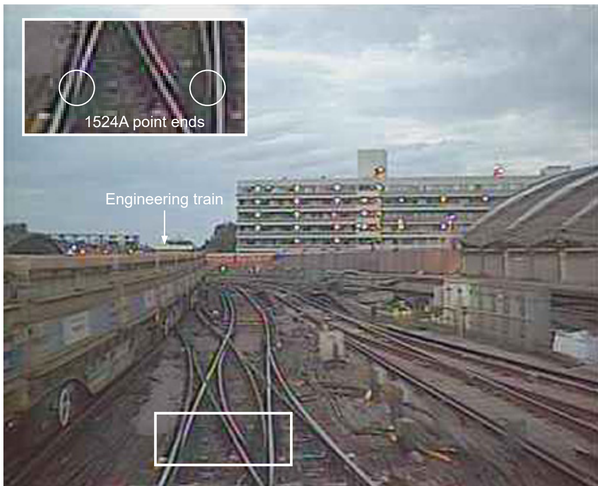
Figure 8: View from the train's forward facing CCTV showing 1524A points lying approximately midway between normal (wide gap at right-hand point end, no gap at left-hand point end) and reverse (gap only at left-hand point end)
