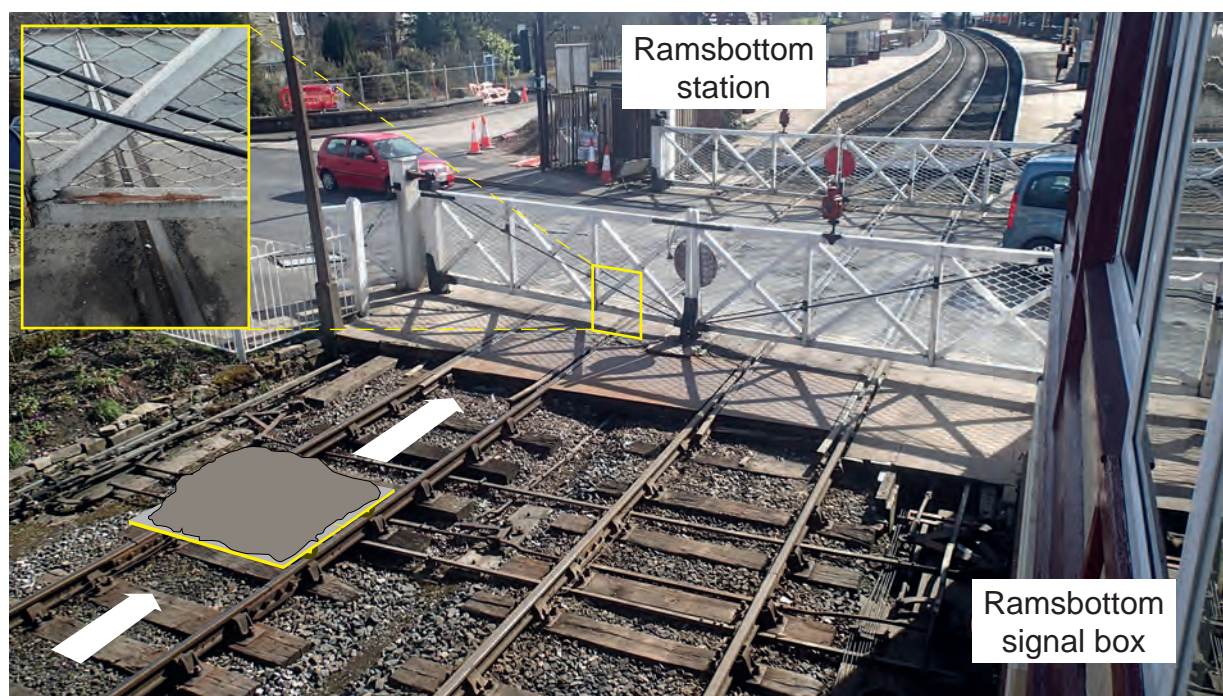
Figure 6: Representation of the trolley striking the level crossing gate (inset image courtesy of East Lancashire Railway)
