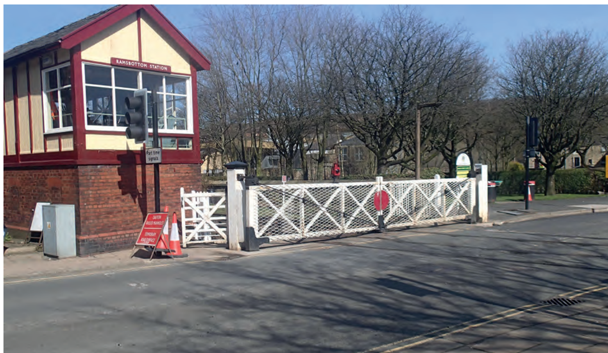
Figure 5: Ramsbottom signal box and level crossing
