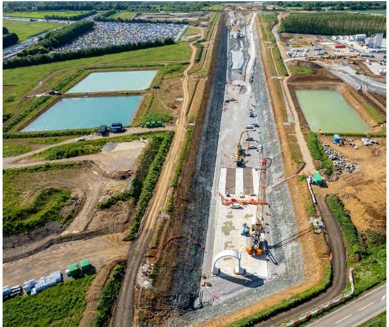
Green tunnel land being prepared for pre-cast concrete segments installation.
