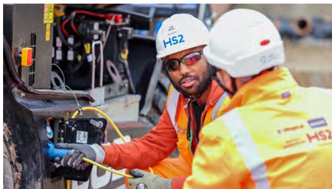
Engineers charging electric plant.
