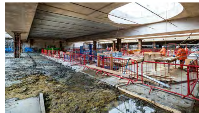
Work has started on the platforms of Old Oak Common station.
