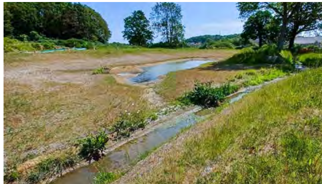
Our work has seen Newyears Green Bourne realigned, with its banks smoothed out and replanted to attract wildlife, © Align.
