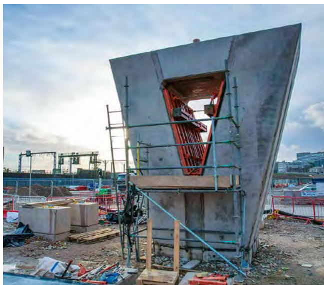
A viaduct support at Curzon Street, Birmingham.
