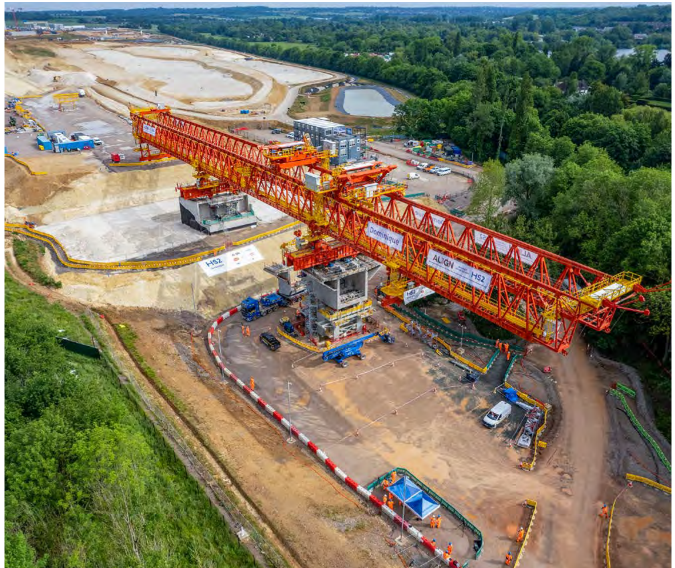
Dominique, the pre-cast concrete launching girder for the Colne Valley viaduct.
