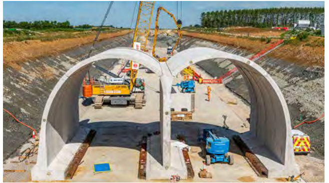
Construction starts on HS2's first 'green tunnel' at Chipping Warden, Northamptonshire.
