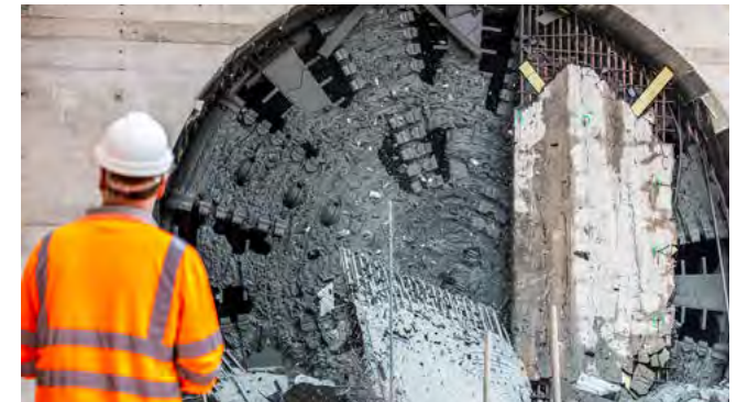
The moment of breakthrough by the tunnel boring machine at Long Itchington Wood.
