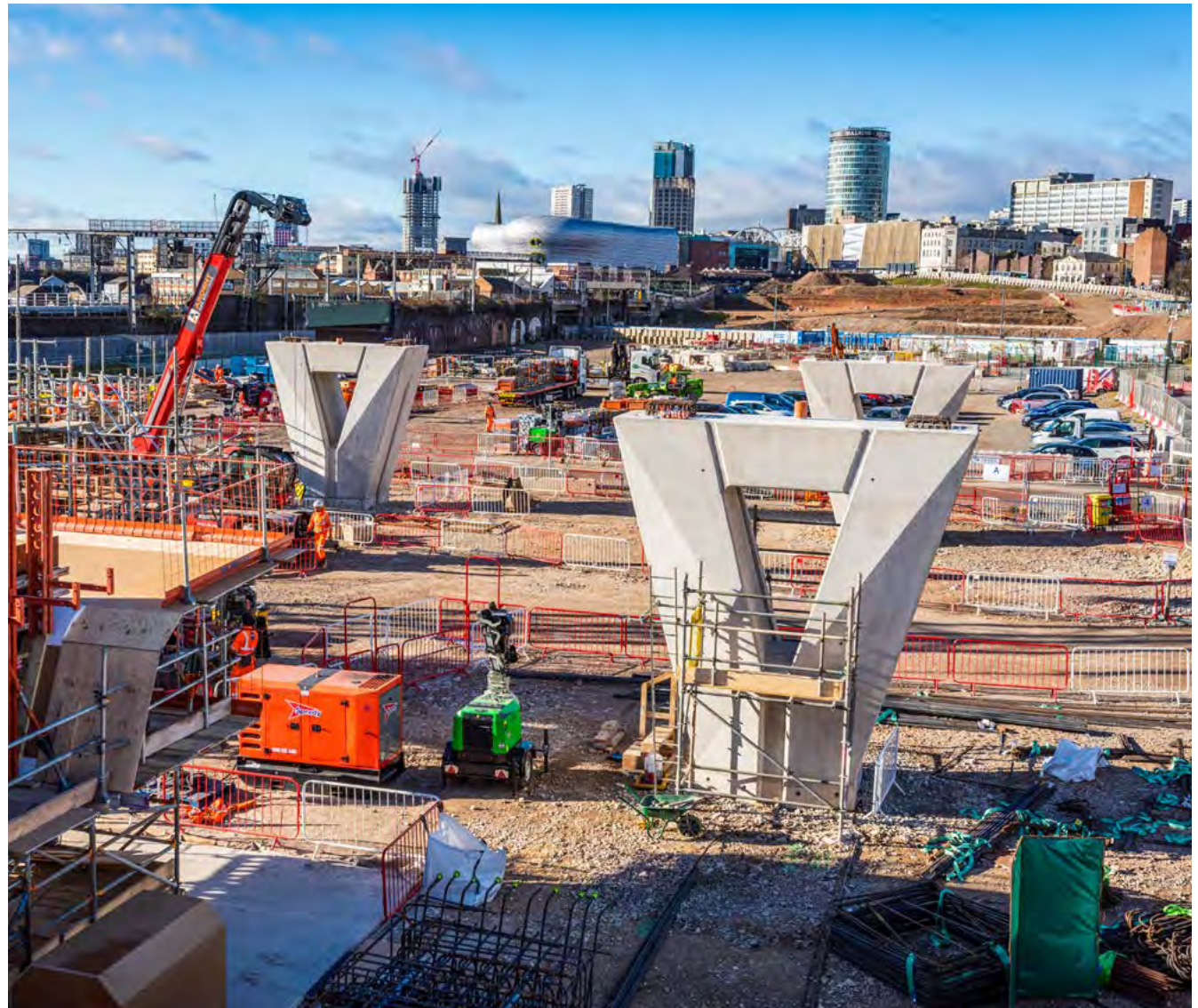
The Curzon Street station work site in Birmingham.
