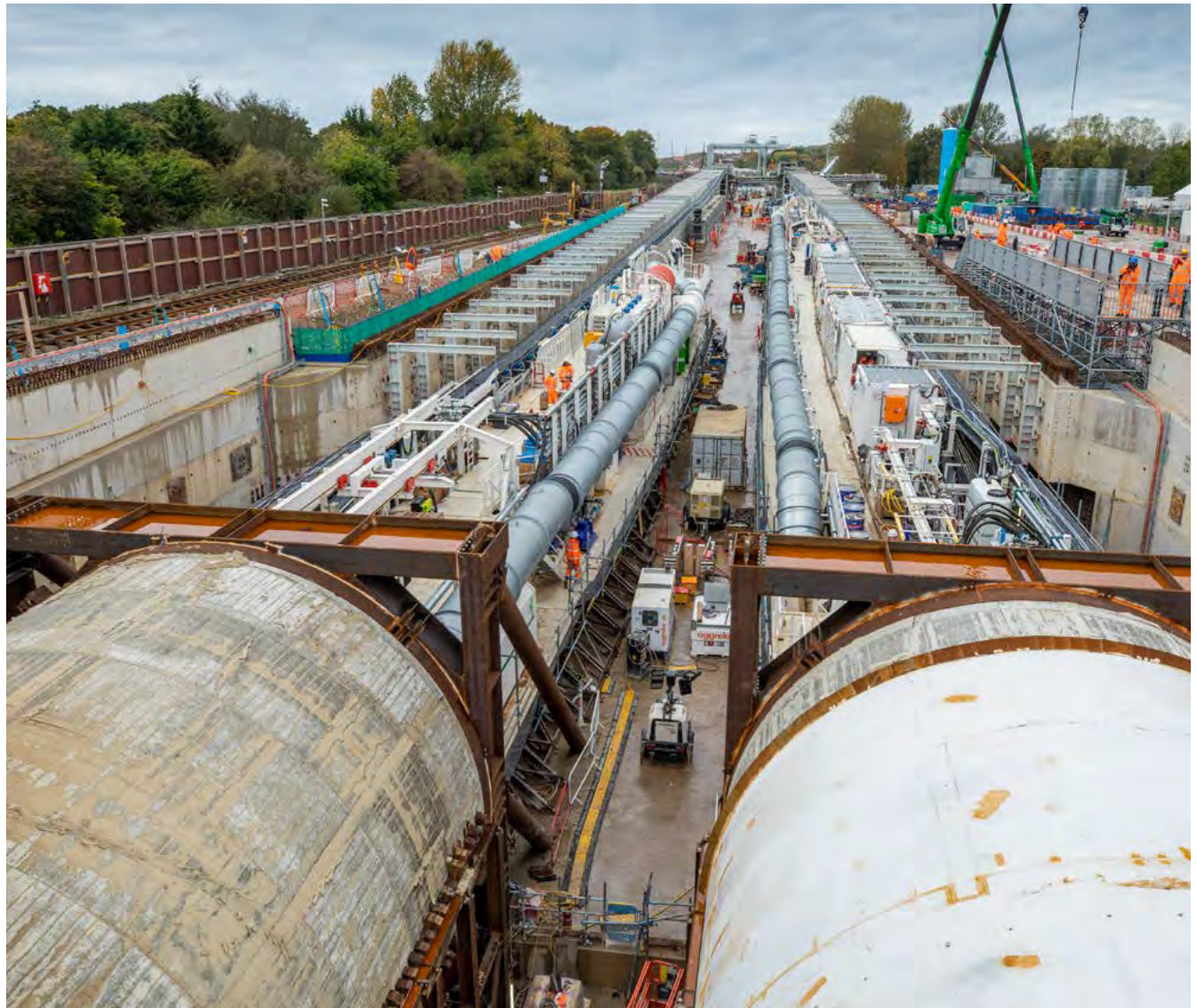
Tunnel boring machines set up for use in London.
