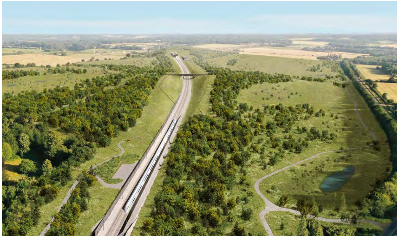
A visualisation of a disguised cutting showing how HS2 trains will be 'hidden' when they run.
