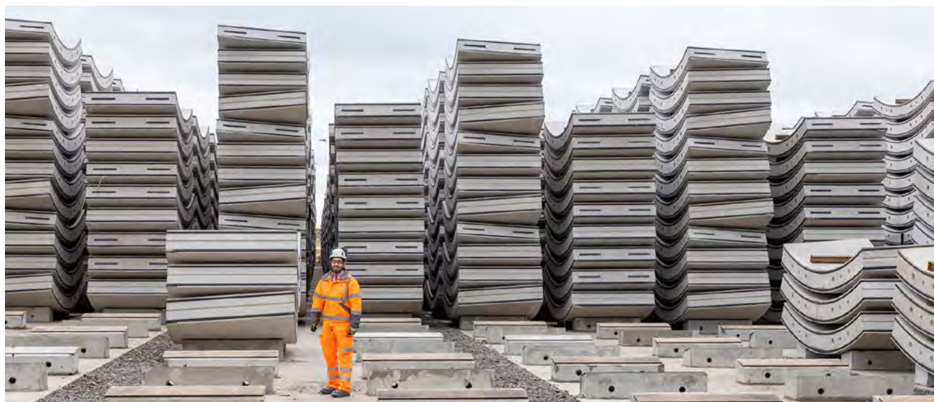
Pre-cast concrete segments laid out ready for use on the Thames Valley viaduct.
