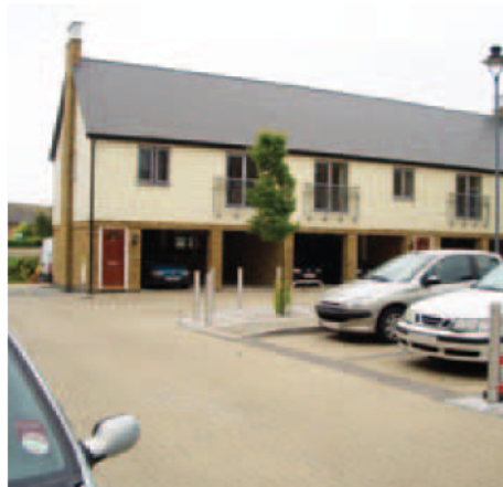
Undercroft parking facing onto central parking court
