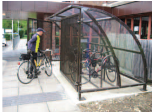
Covered shelter secured with lockable gates
