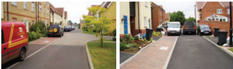
Examples of shared surfaces which are not appropriate for the location, note the indiscriminate parking
