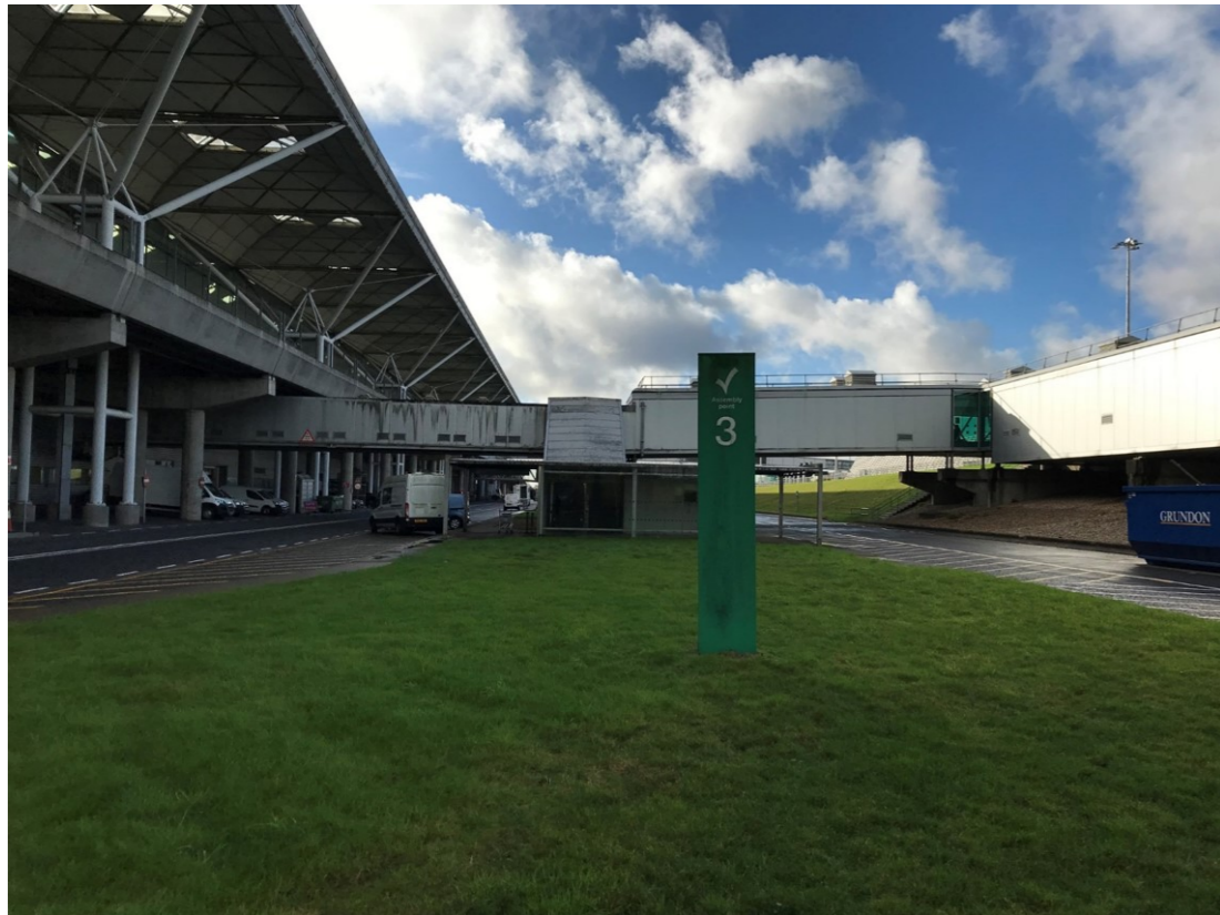
1 - VIEW OF TERMINAL AND SAT 3 CONNECTION
