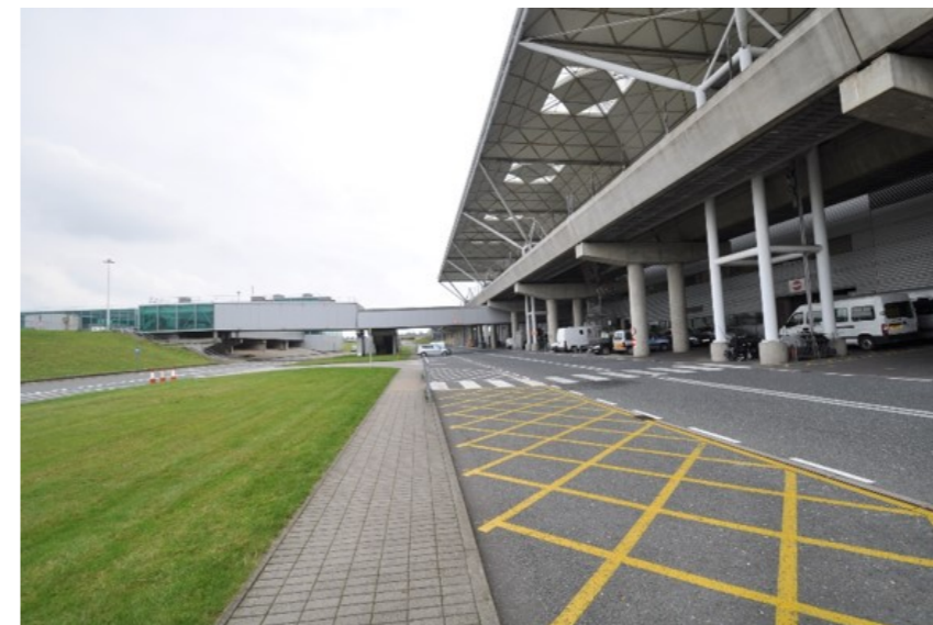
4 - VIEW OF TERMINAL AND SAT 3 CONNECTION
