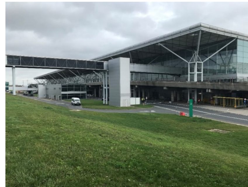
3 - VIEW OF TERMINAL AND SAT 2 CONNECTION
