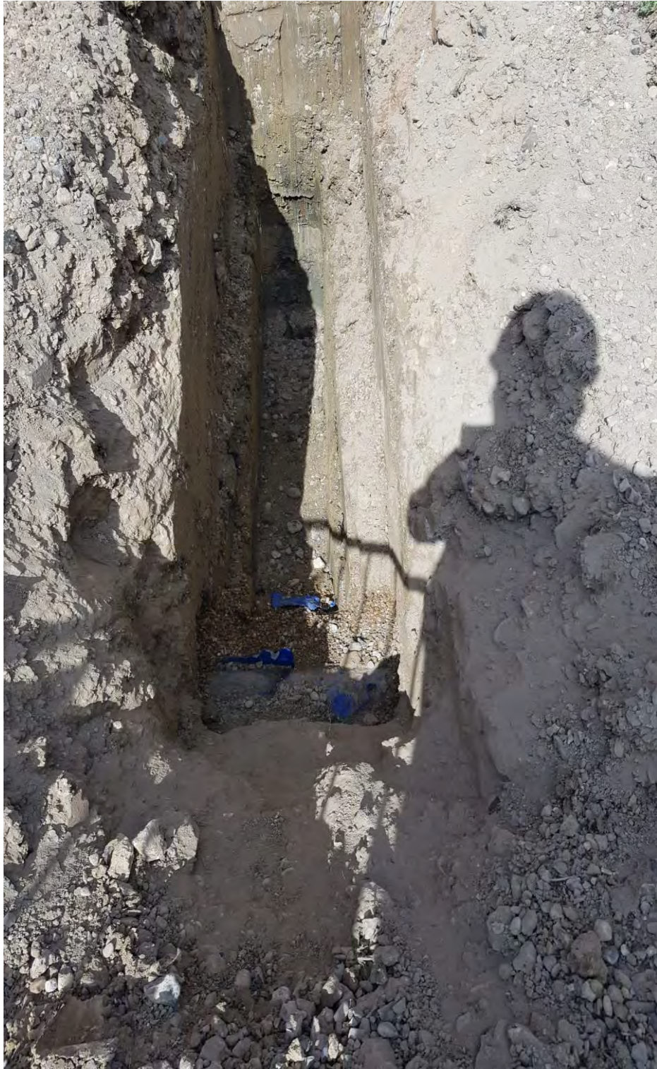
RC04 GL to 1.50m Inspection Pit
