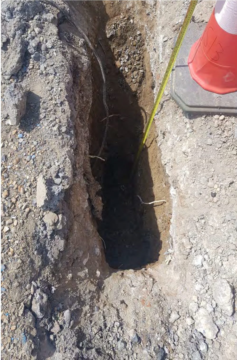
DS13 GL to 1.50m Inspection Pit
