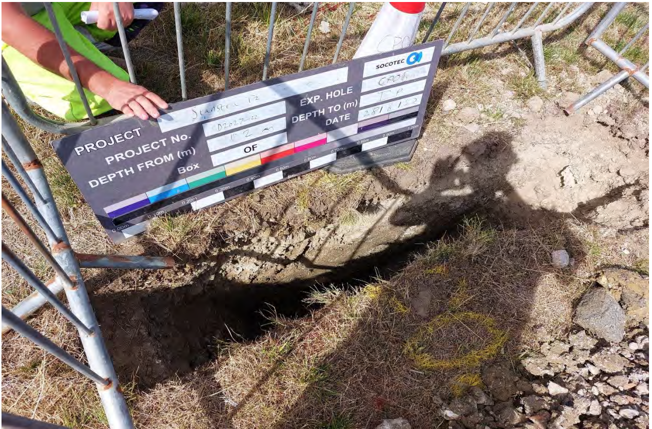
CP06 GL to 1.50m Inspection Pit
