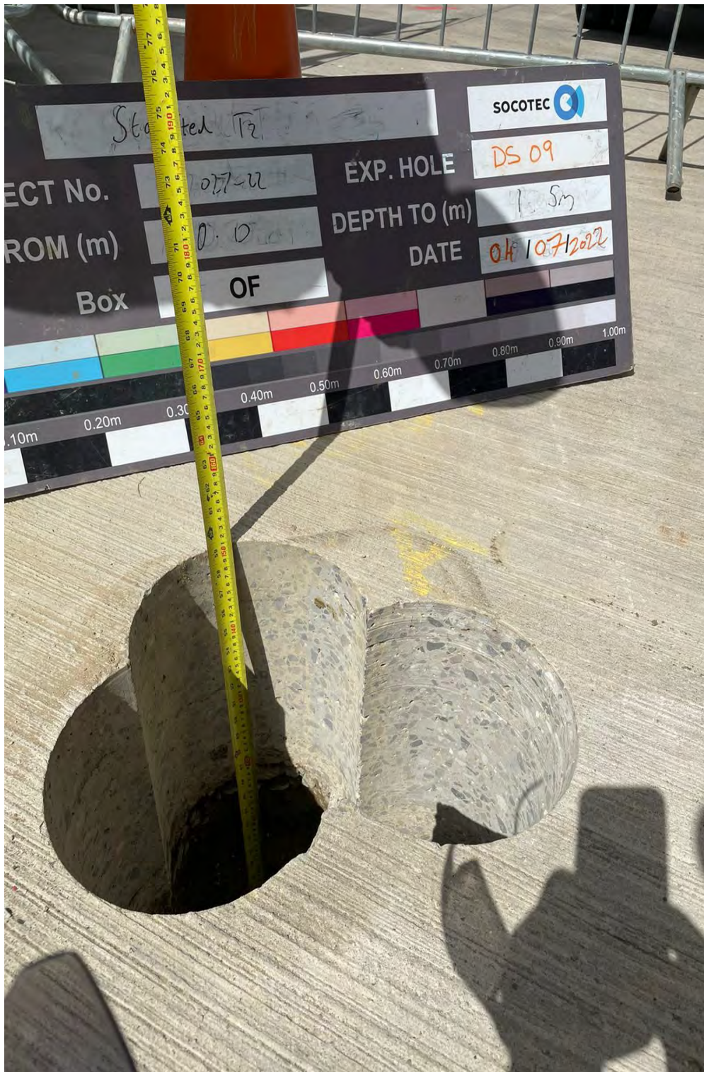
DS09 GL to 1.50m Inspection Pit
