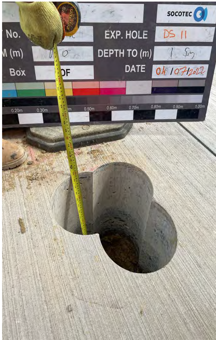
DS11 GL to 1.50m Inspection Pit
