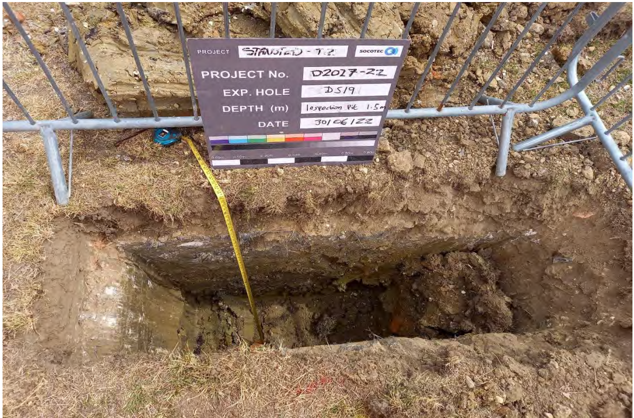
DS19 GL to 1.50m Inspection Pit
