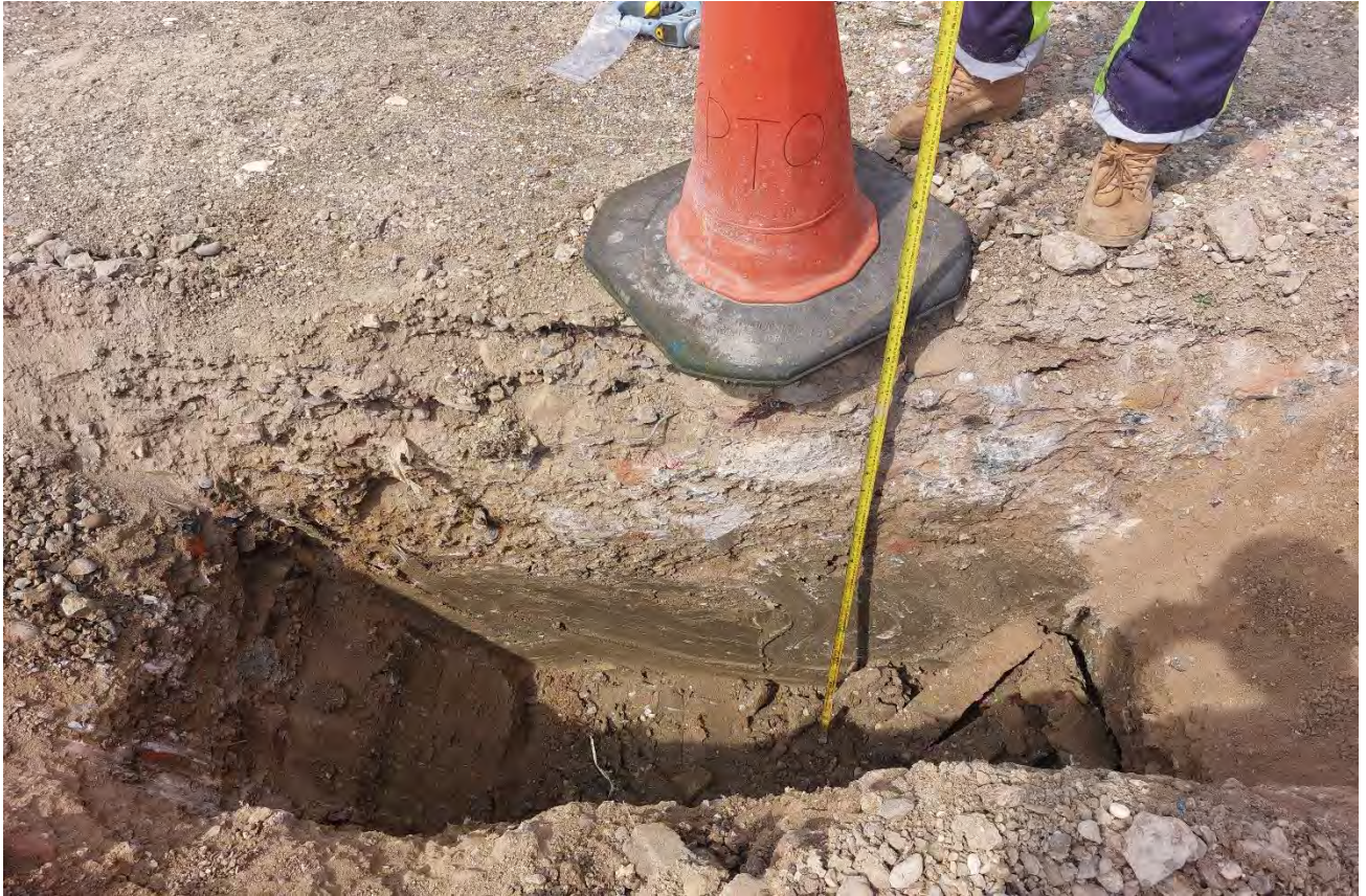
CPT03 GL to 1.50m Inspection Pit
