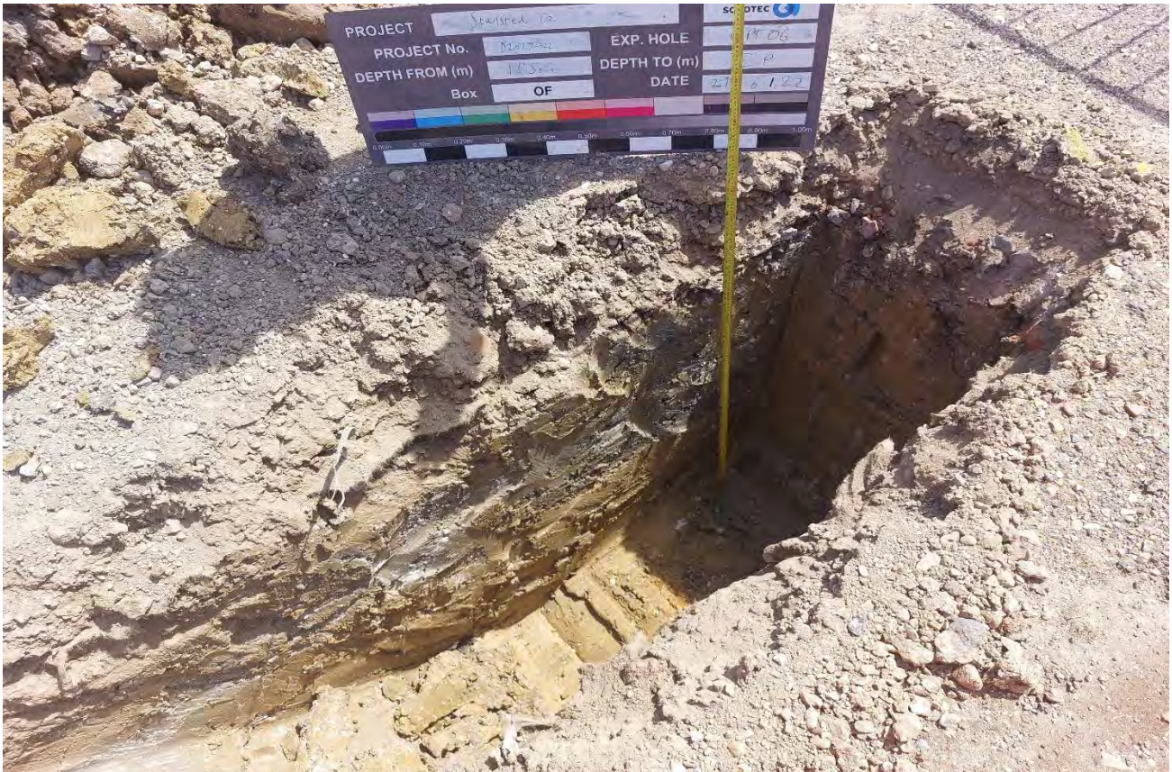
CPT06 GL to 1.50m Inspection Pit
