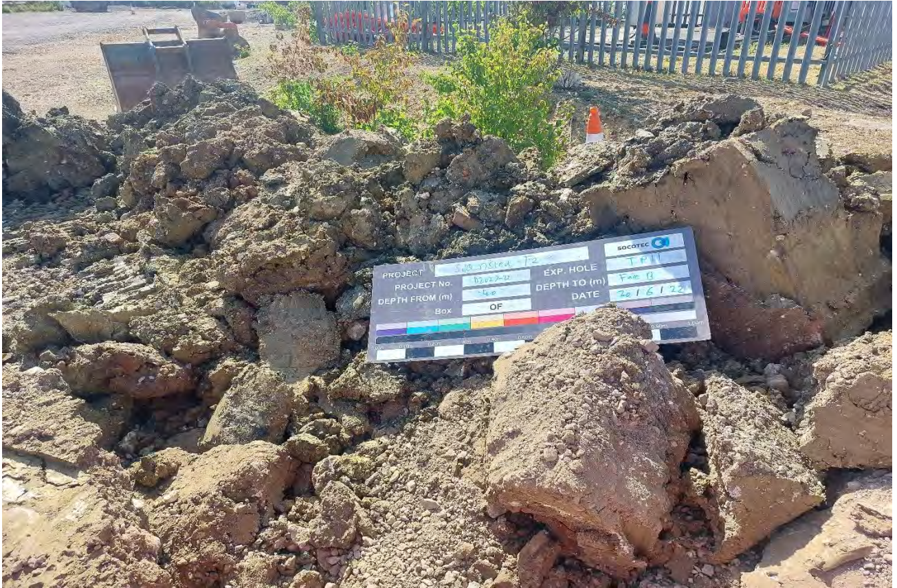
TP11 GL to 4.00m Spoil
