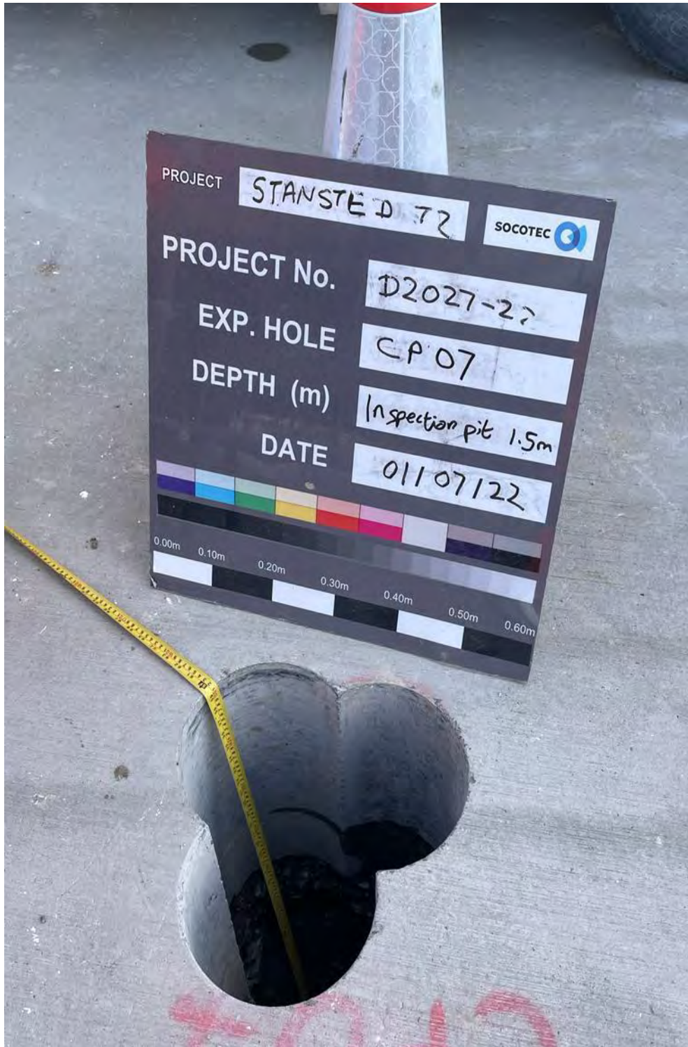
CP07 GL to 1.50m Inspection Pit
