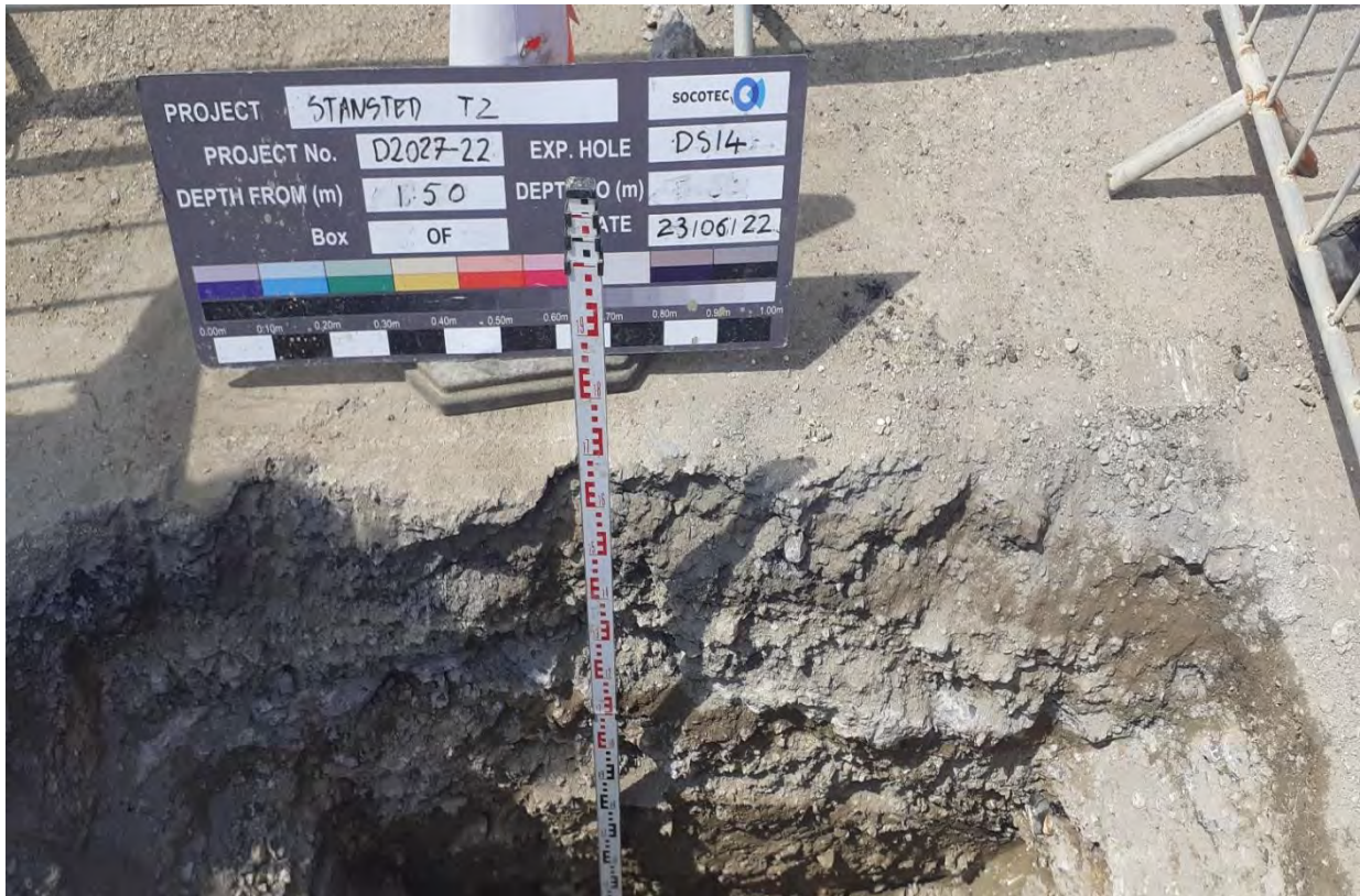
DS14 GL to 1.50m Inspection Pit
