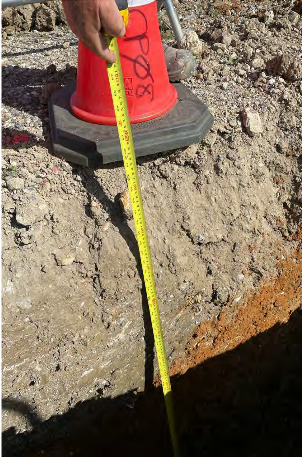
CP08 GL to 1.50m Inspection Pit
