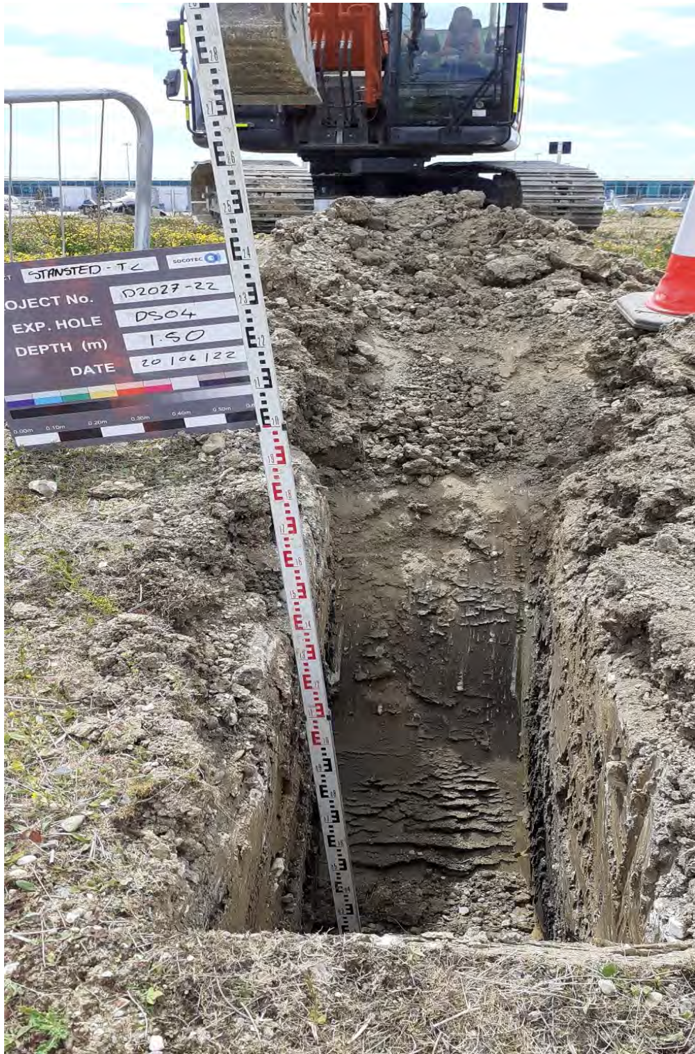
DS04 GL to 1.50m Inspection Pit
