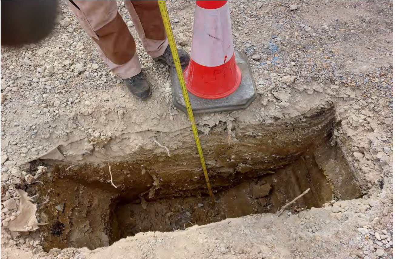
CPT12 GL to 1.50m Inspection Pit
