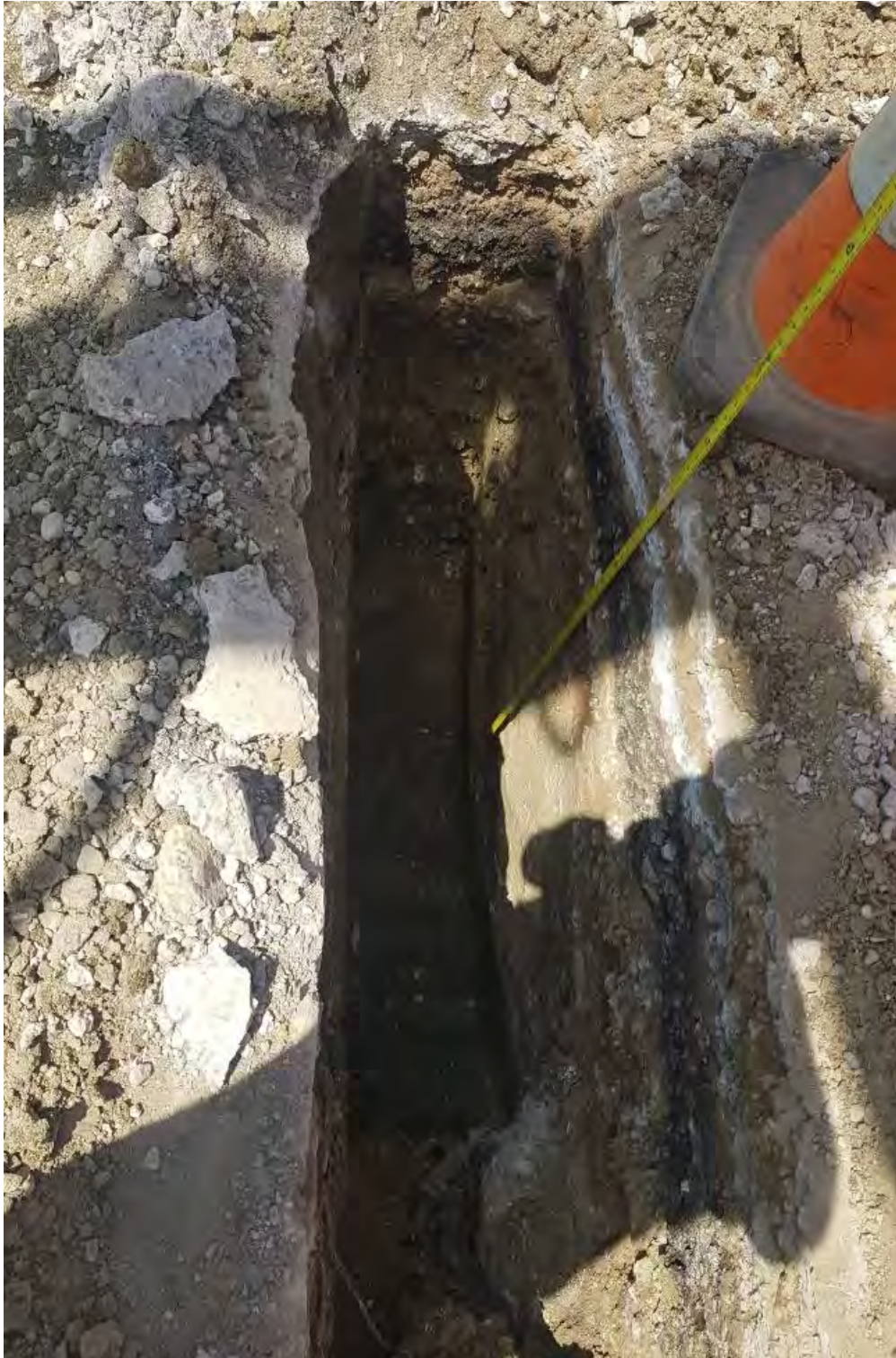
DS05 GL to 1.50m Inspection Pit
