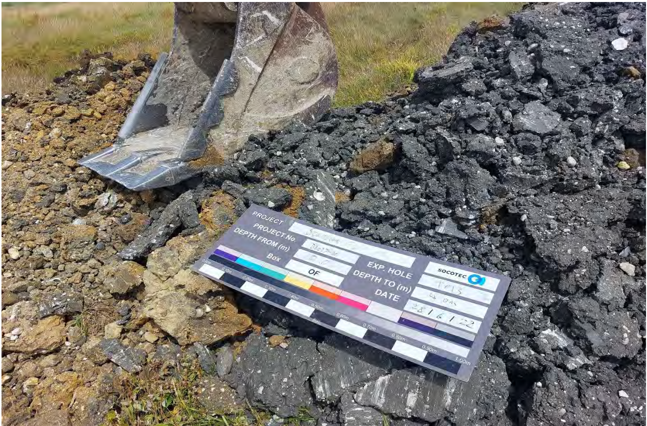
TP13 GL to 4.00m Spoil
