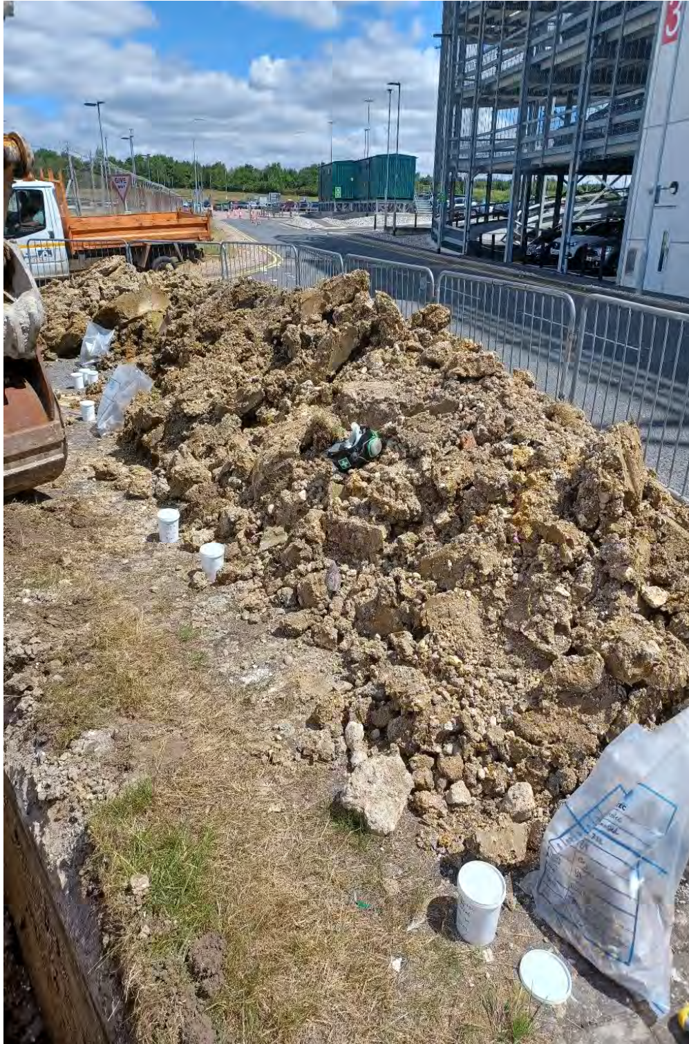
TP12 GL to 4.00m Spoil
