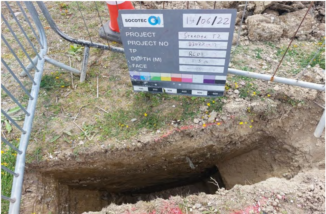
RC01 GL to 1.50m Inspection Pit
