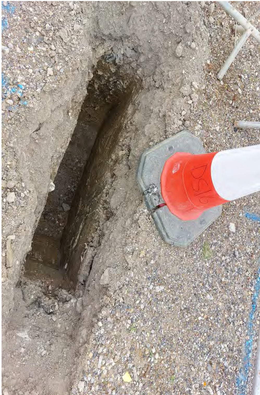
DS16 GL to 1.50m Inspection Pit
