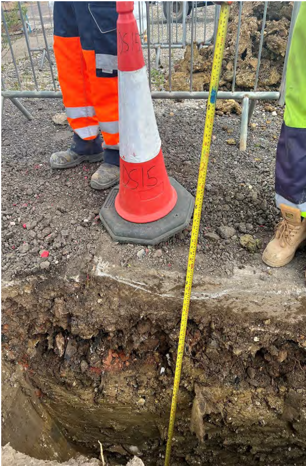
DS15 GL to 1.50m Inspection Pit
