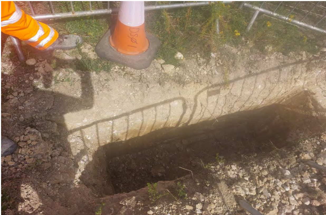
DS01 GL to 1.50m Inspection Pit
