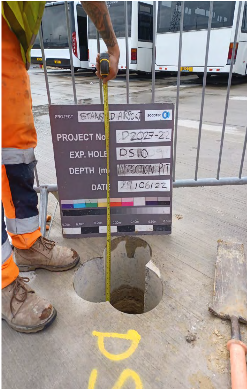
DS10 GL to 1.50m Inspection Pit
