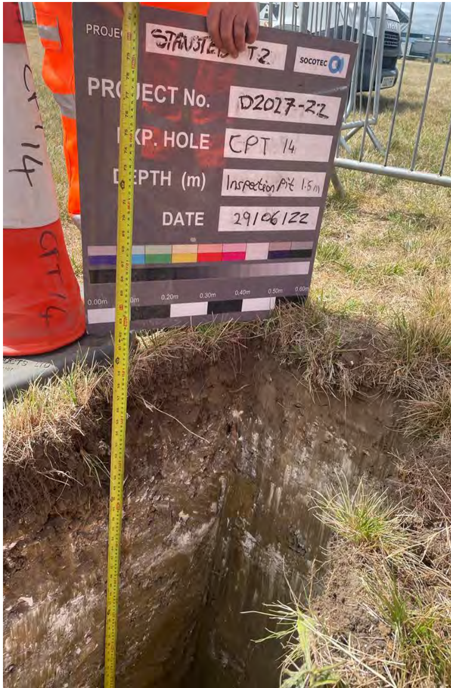
CPT14 GL to 1.50m Inspection Pit
