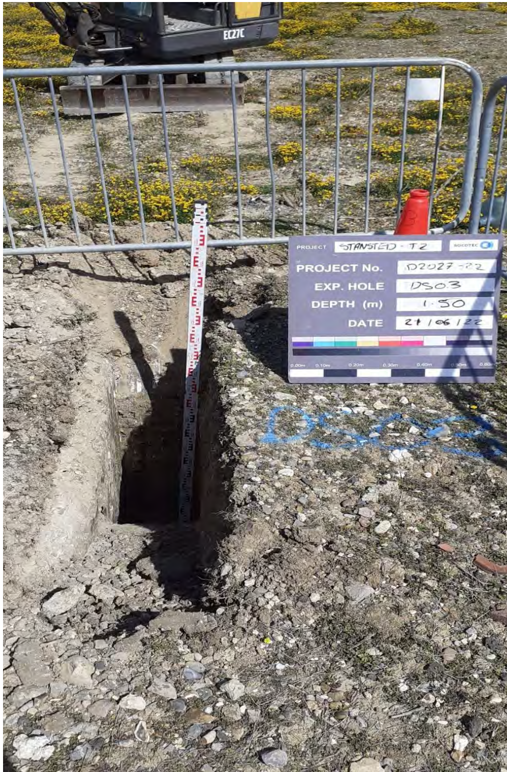
DS03 GL to 1.50m Inspection Pit
