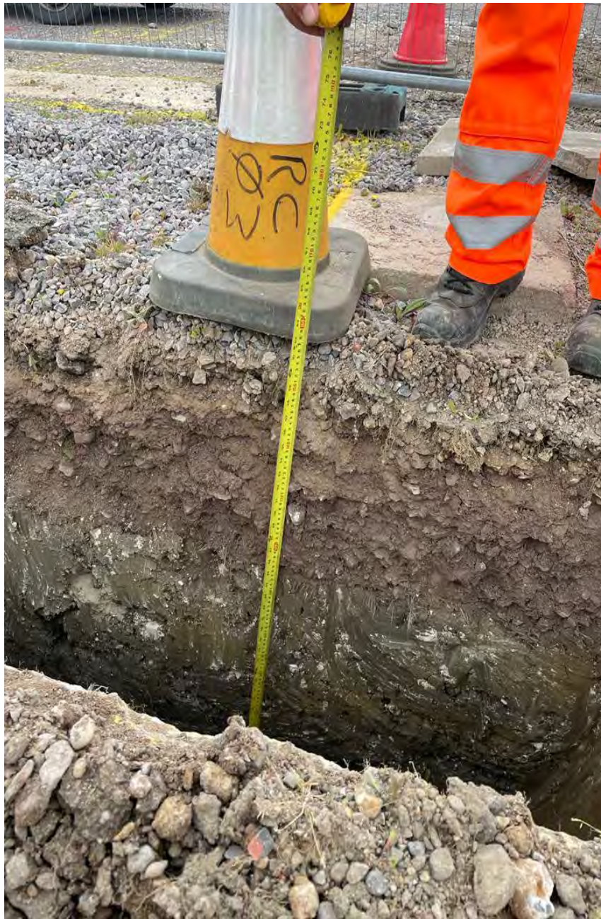
RC03 GL to 1.50m Inspection Pit
