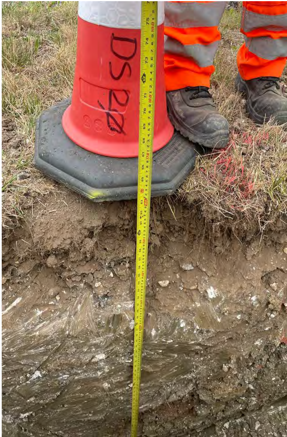
DS20 GL to 1.50m Inspection Pit
