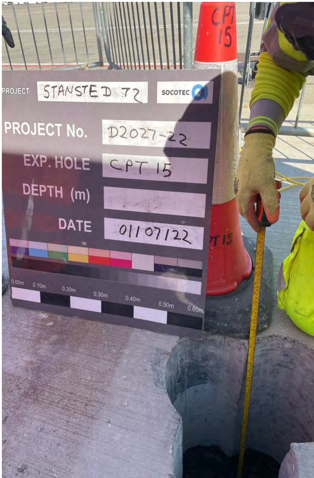
CPT15 GL to 1.50m Inspection Pit
