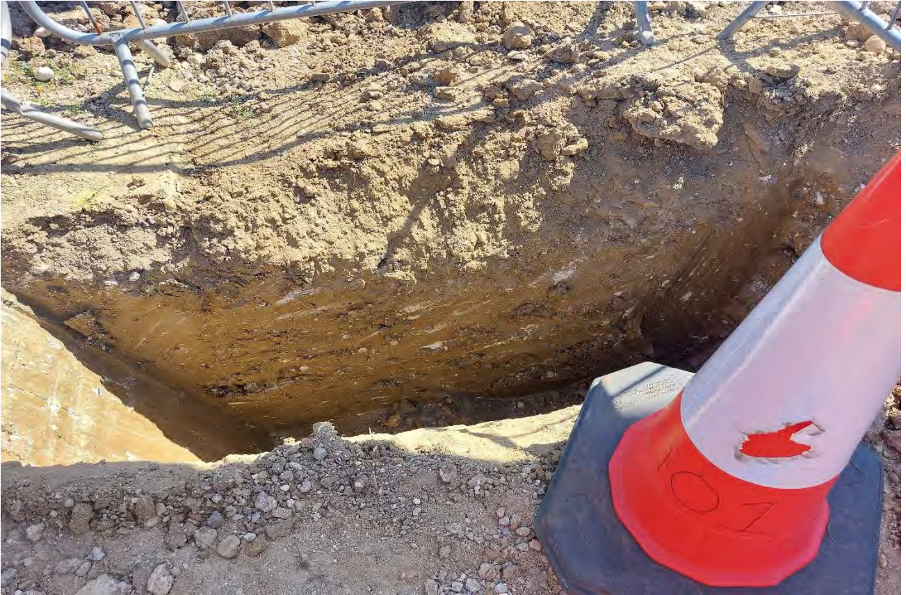
CPT01 GL to 1.50m Inspection Pit
