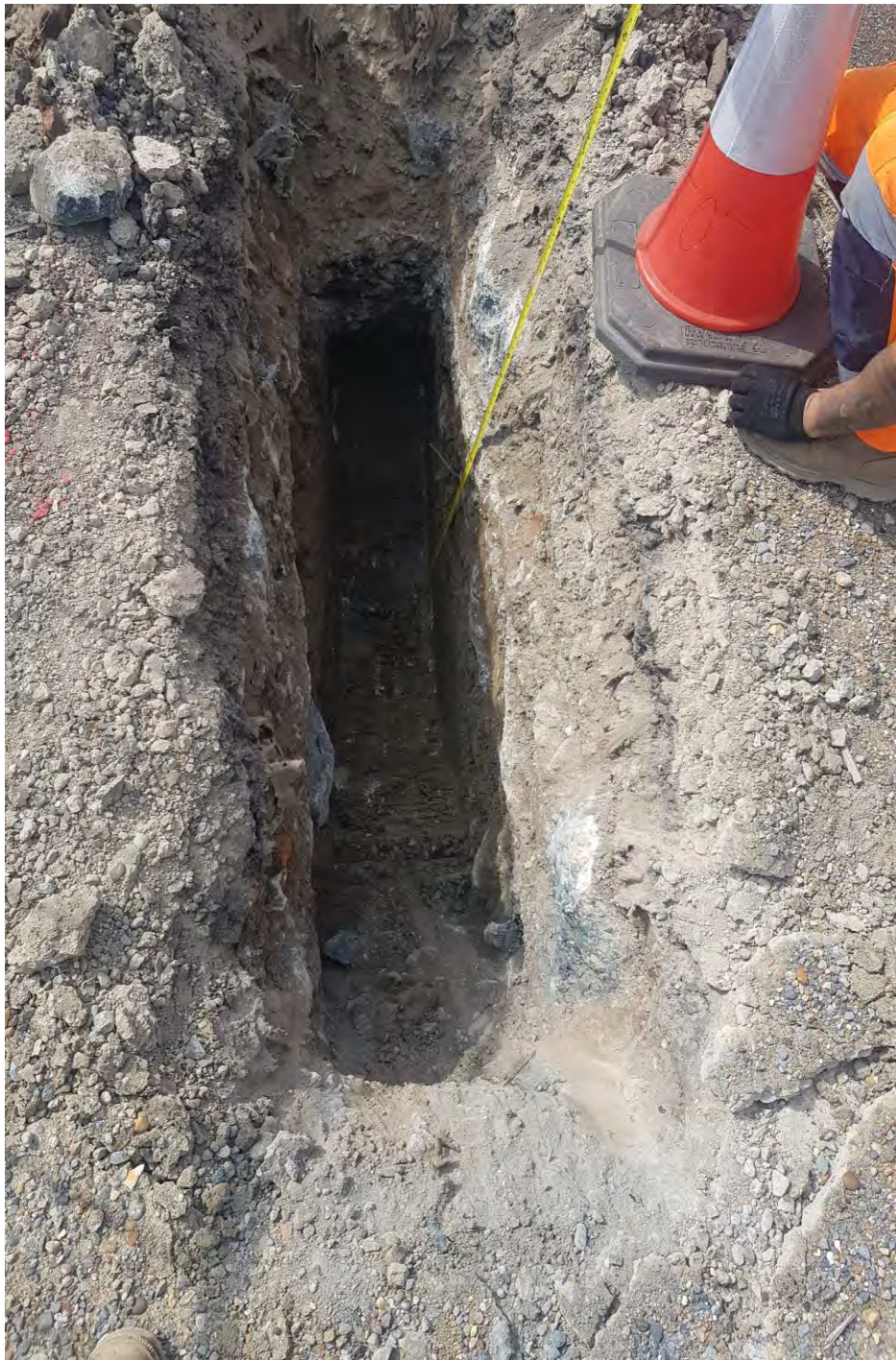
CPT07 GL to 1.50m Inspection Pit
