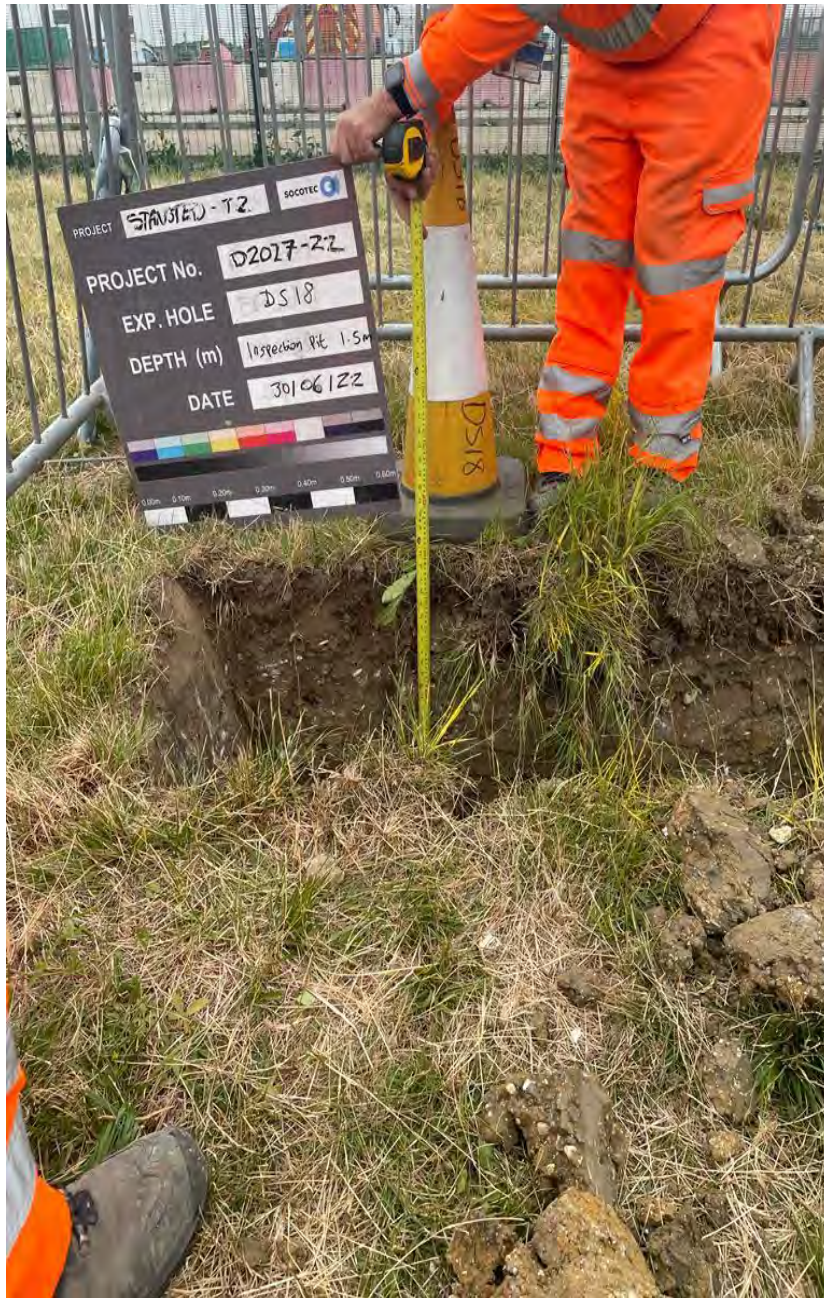
DS18 GL to 1.50m Inspection Pit
