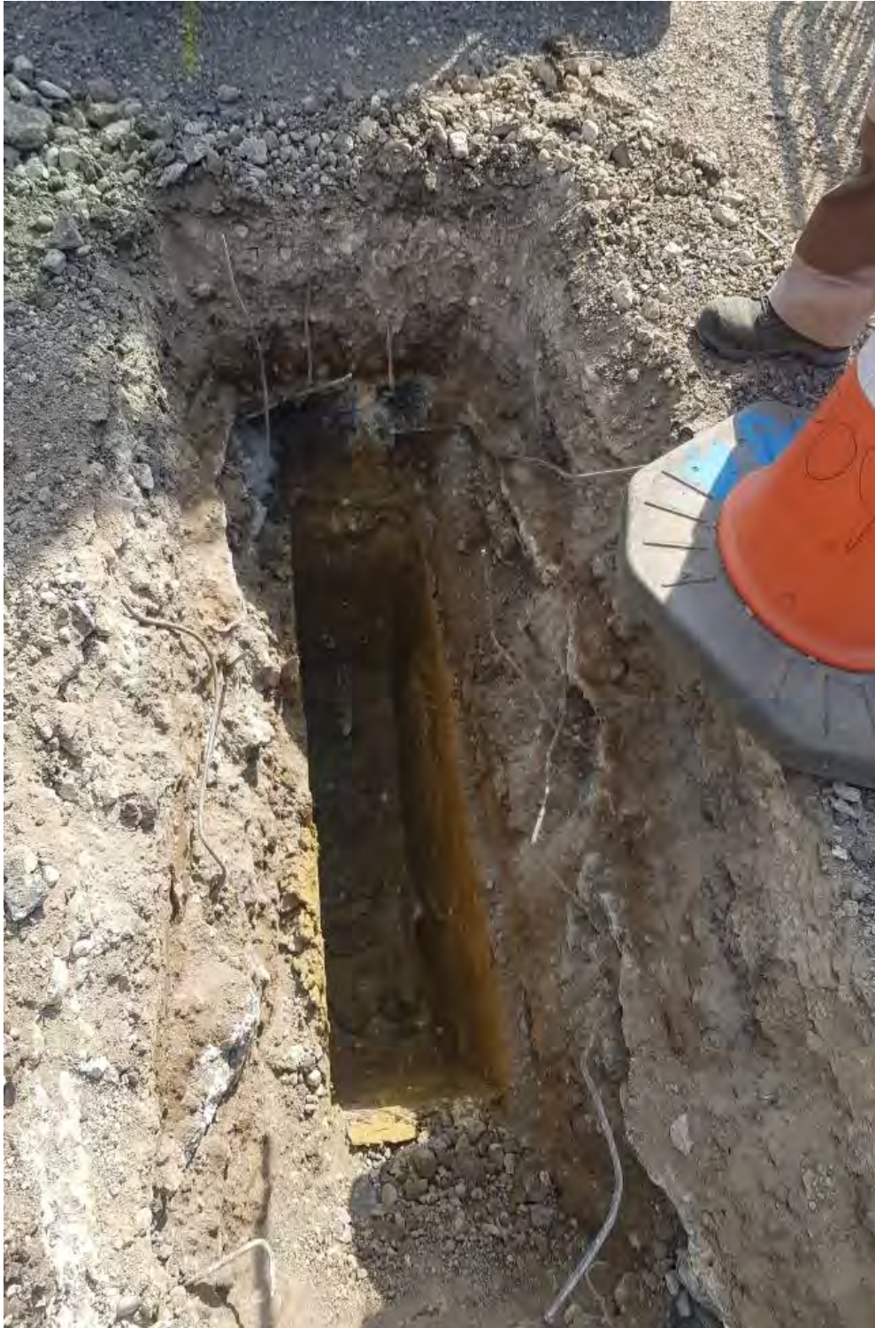
CP09 GL to 1.50m Inspection Pit
