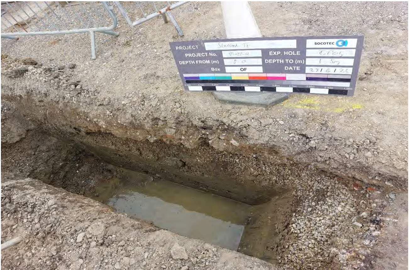
CP05 GL to 1.50m Inspection Pit
