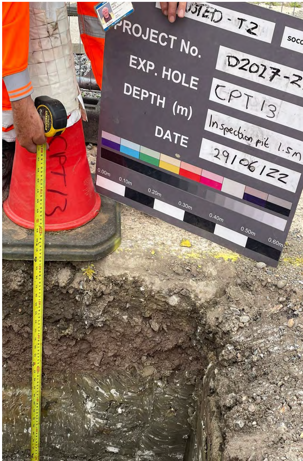
CPT13 GL to 1.50m Inspection Pit
