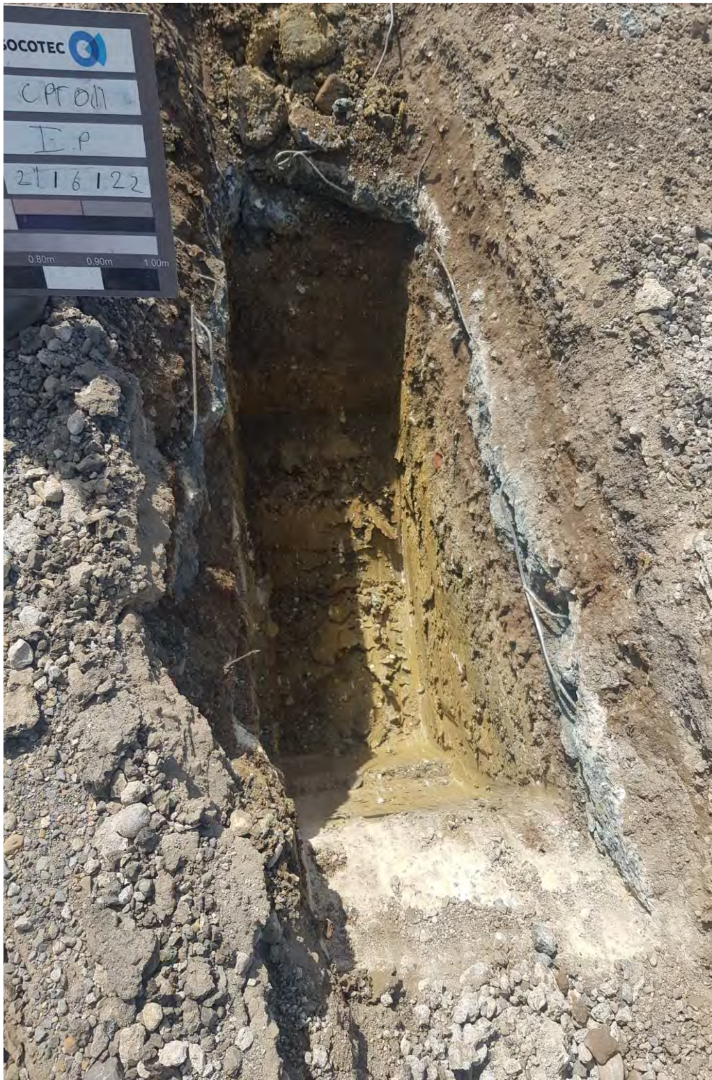
CPT11 GL to 1.50m Inspection Pit
