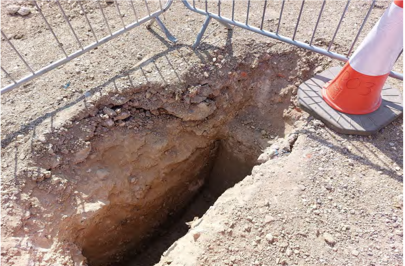
CP03 GL to 1.50m Inspection Pit
