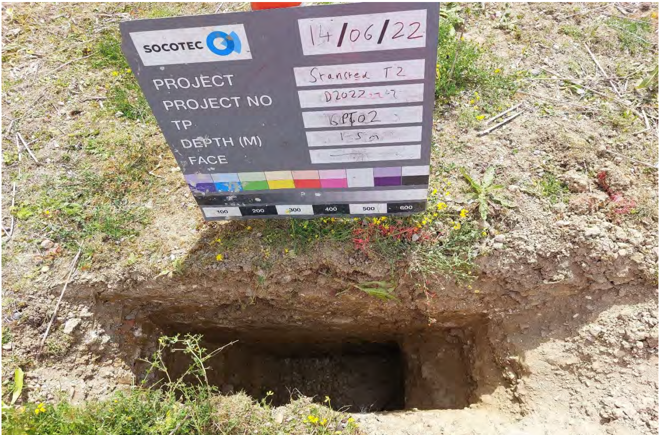
CPT02 GL to 1.50m Inspection Pit
