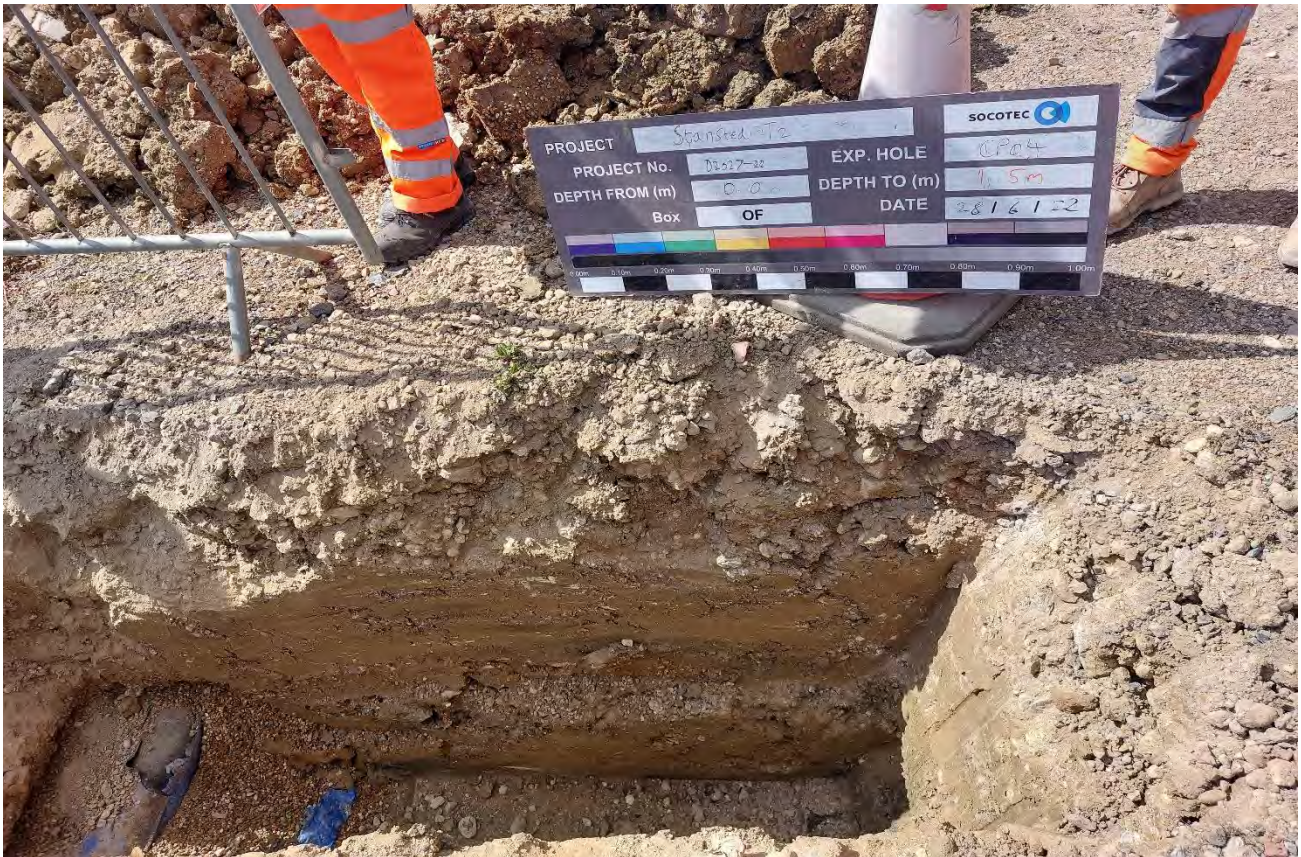
CP04 GL to 1.50m Inspection Pit
