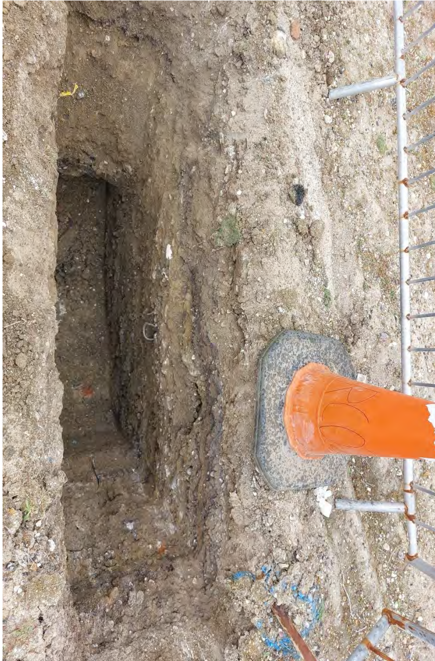
RC02 GL to 1.50m Inspection Pit
