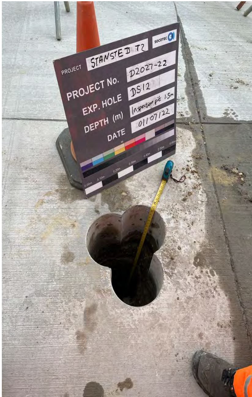
DS12 GL to 1.50m Inspection Pit
