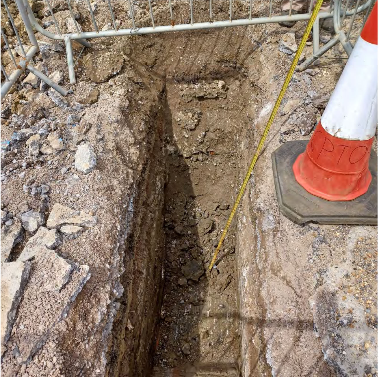
CPT05 GL to 1.50m Inspection Pit
