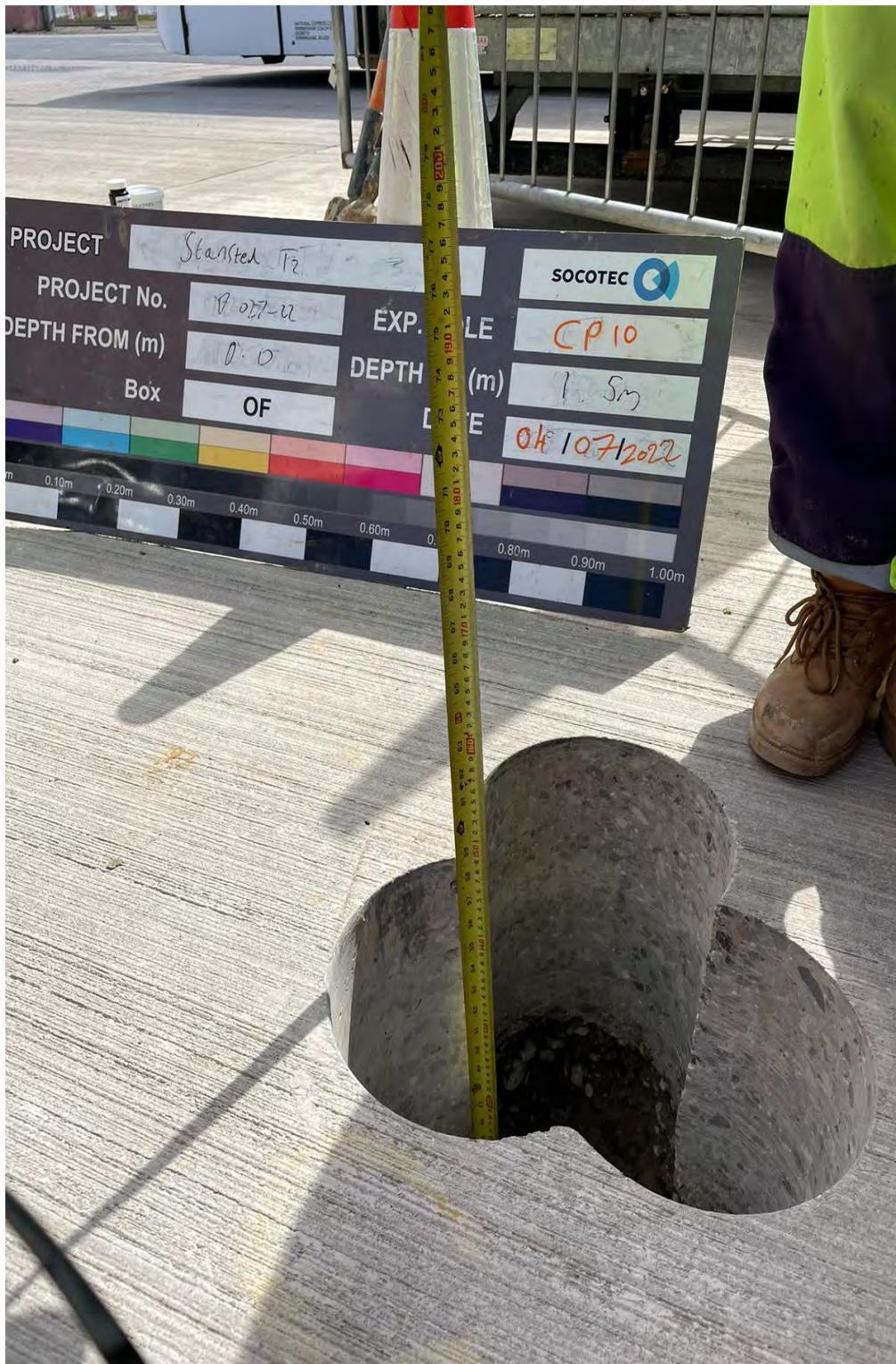
CP10 GL to 1.50m Inspection Pit
