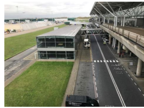
Existing Terminal and Bus-gate Building
