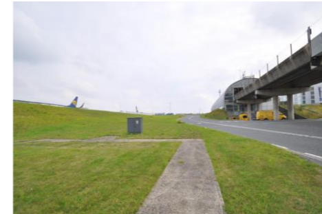
Existing Track Transit System Maintenance Building
