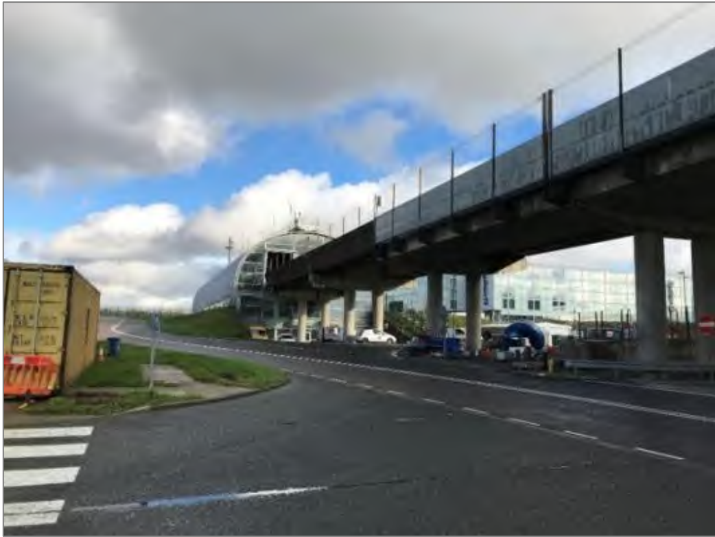
Photograph 3: View northeast towards TTS Maintenance
