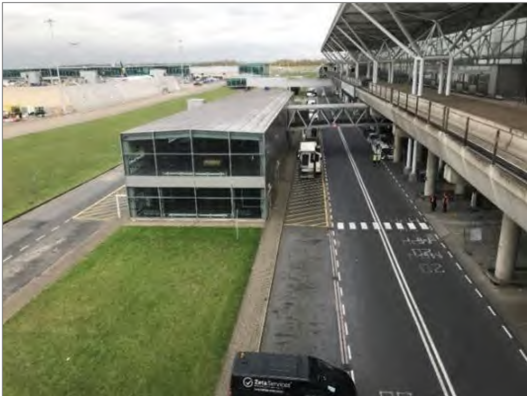
Photograph 6: View northeast towards Terminal 1 and APV
