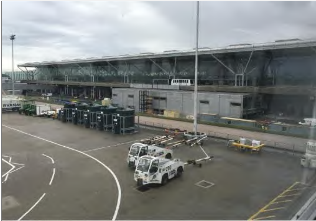
Photograph 5: View southeast towards Terminal 1 from Apron and APV
