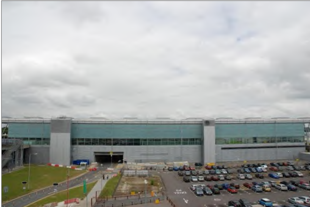
Photograph 8: View northeast towards western façade of Terminal 1
