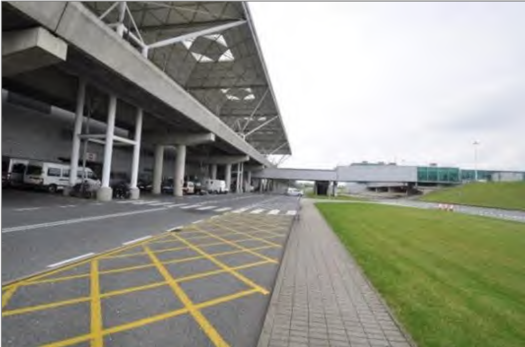
Photograph 4: View northeast towards Terminal 1 and Sat 3 Connection
