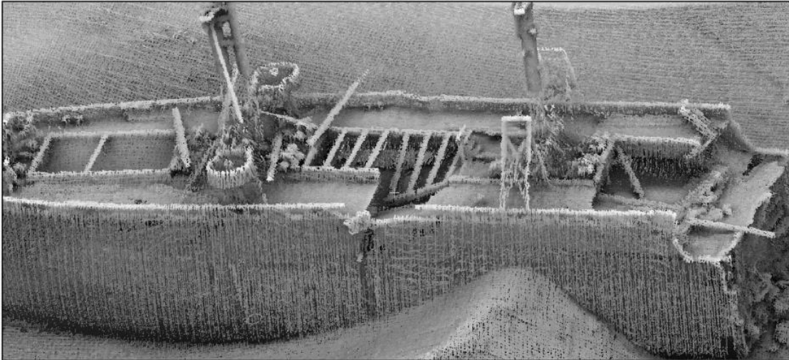
Figure 21 Crack in Hull (ID04) and collapsed upper deck (ID08) overview in the 2020 dataset.
