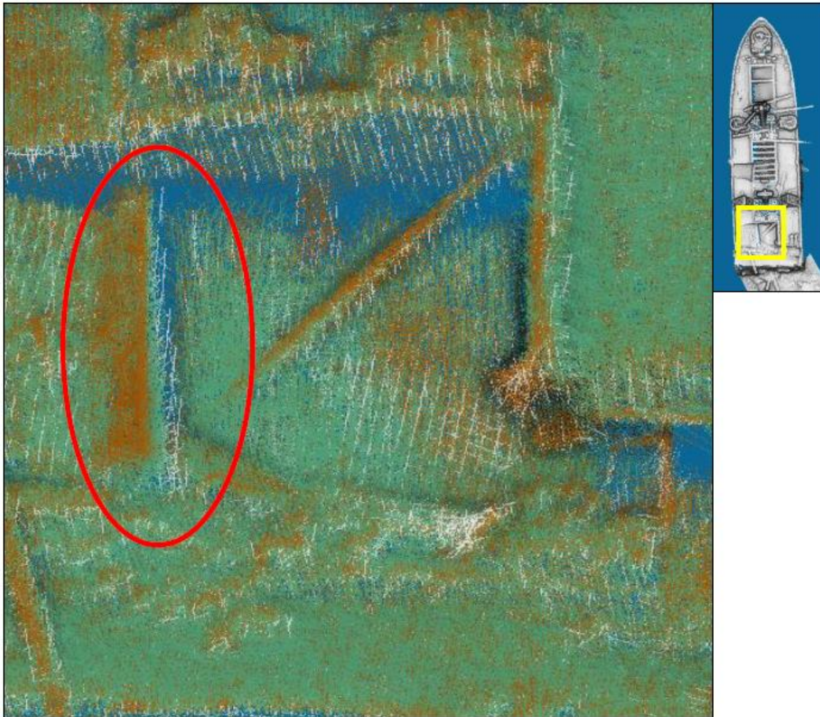
Figure 17 No.3 hatch showing movement of hatch coaming. Brown 2017, green 2019, white 2020.
