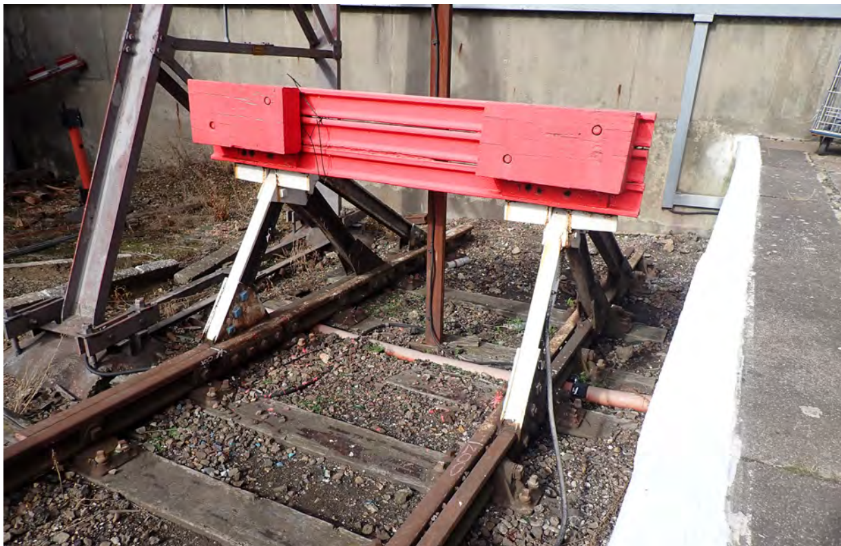
Figure 4: Type of buffer stop at Enfield Town station (platform 3 shown)
