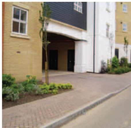
Undercroft secure parking (gated entry).
