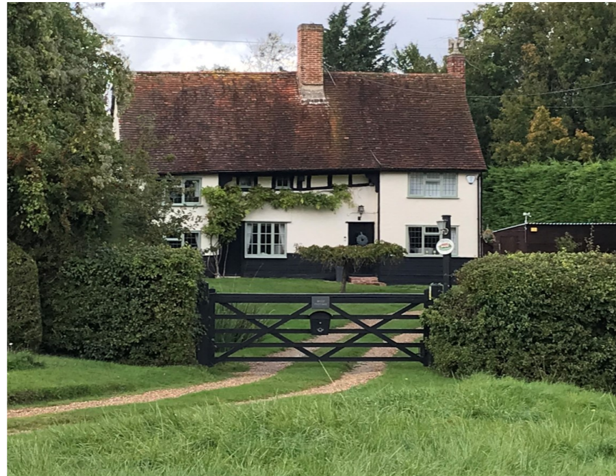
Figure 18 Moat Cottage (source RPS photograph)
