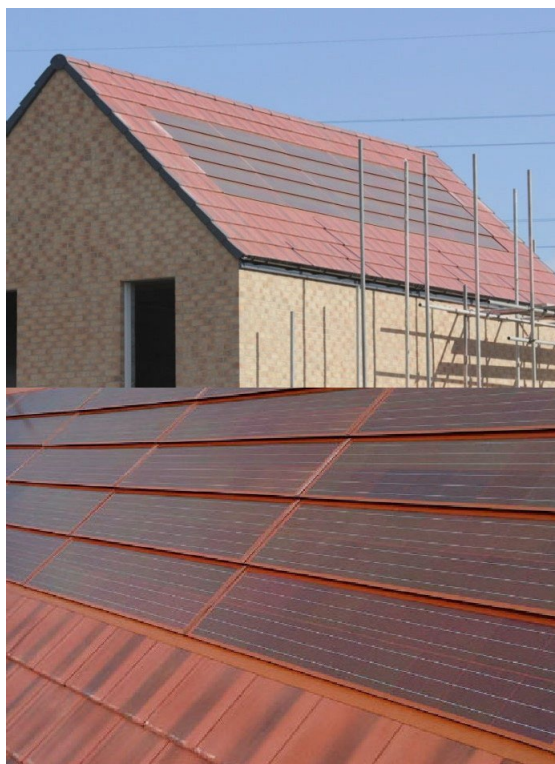
Integrated photovoltaic clay-type roof tile (source: Romag)
