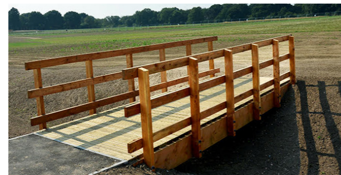
New Timber bridge to ditch crossing improving access onto PRow 48_41
