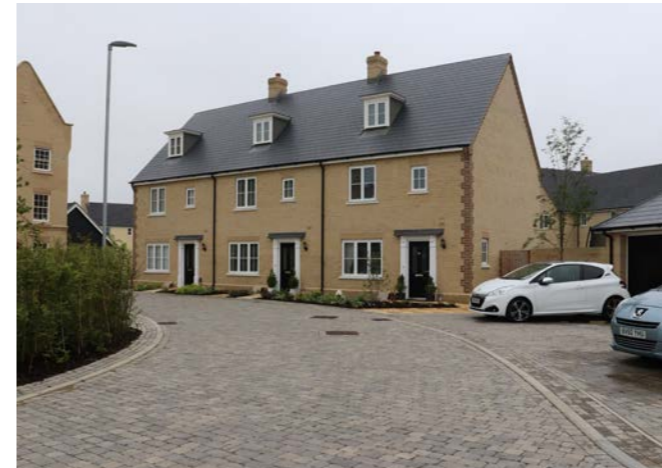
Block paving to shared surfaces
