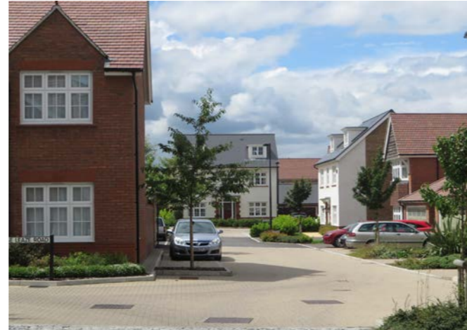
Permeable block paving to parking courts
