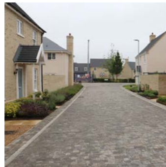
Block paving to shared surfaces
