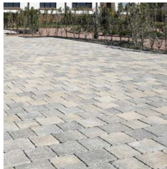
Permeable block paving
