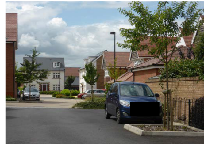
Brick walls to plot boundaries facing parking courts
