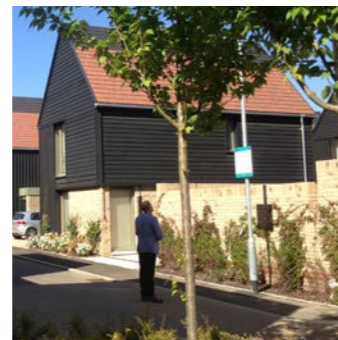
Brick wall to boundary complementing architecture
