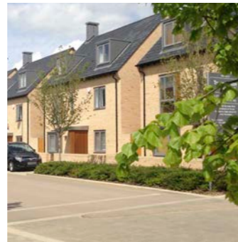
Block paving to raised tables
