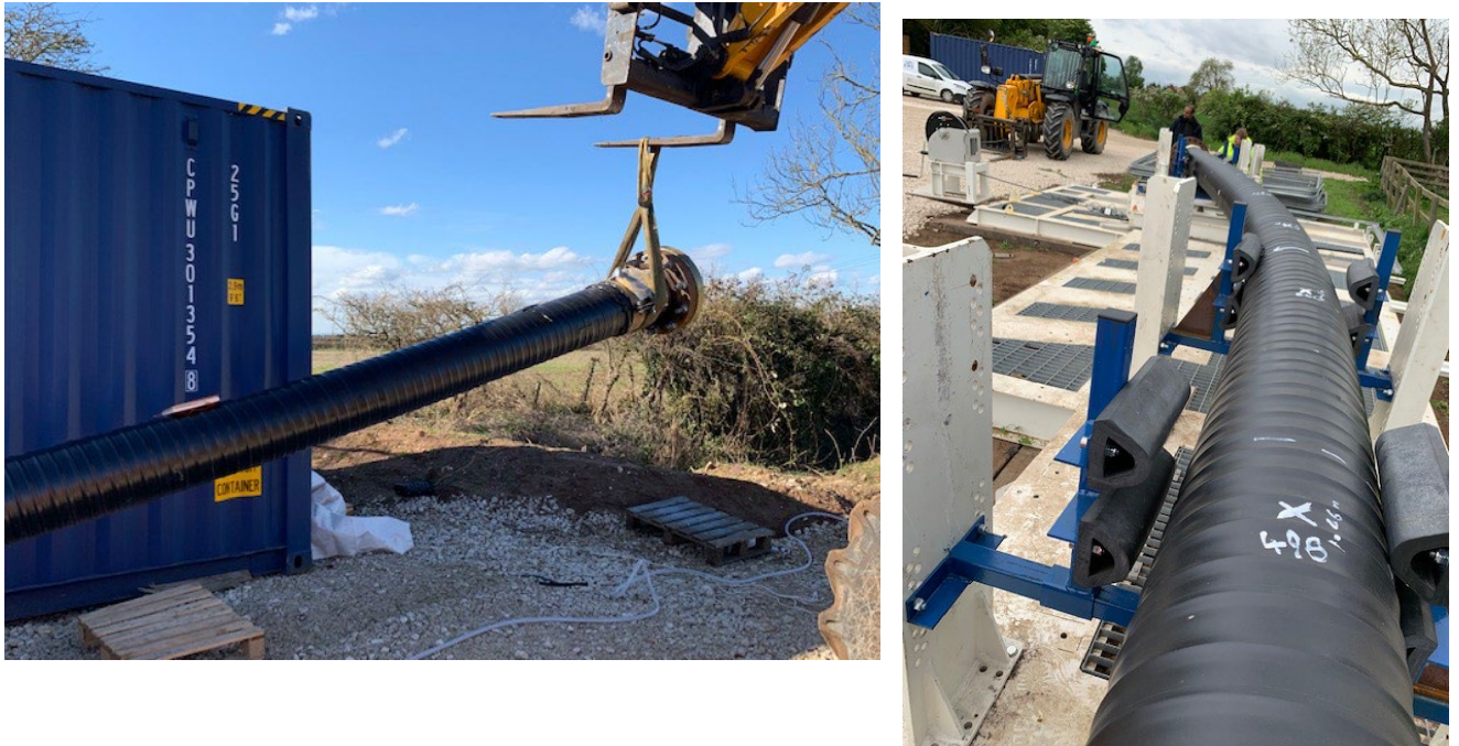
Figure 6-2 - Pipe bending and handling tests using 10m pipe section
