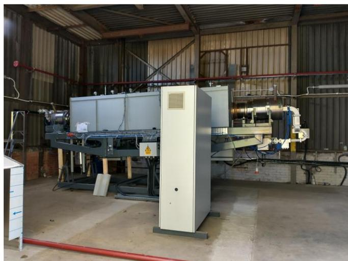
FIG. 29: ROTARY KILN FURNACE DURING INSTALLATION
