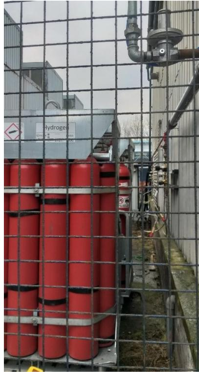
Figure 8. Gas bottle pack in situ supplying Rotary Reduction Furnace, Materials Processing Institute.
