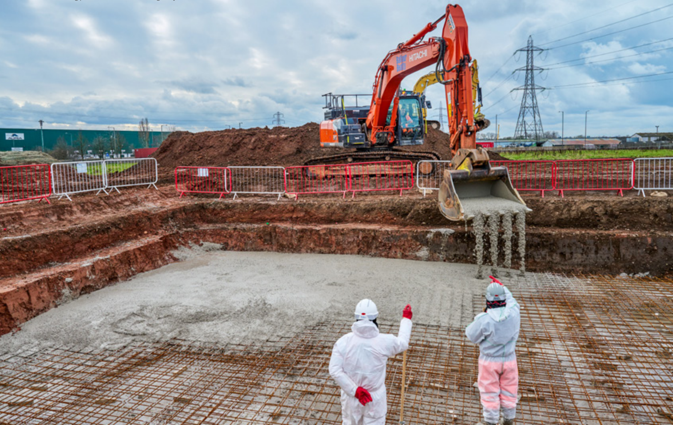
Concrete being poured over rebar at a Kingsbury site.
