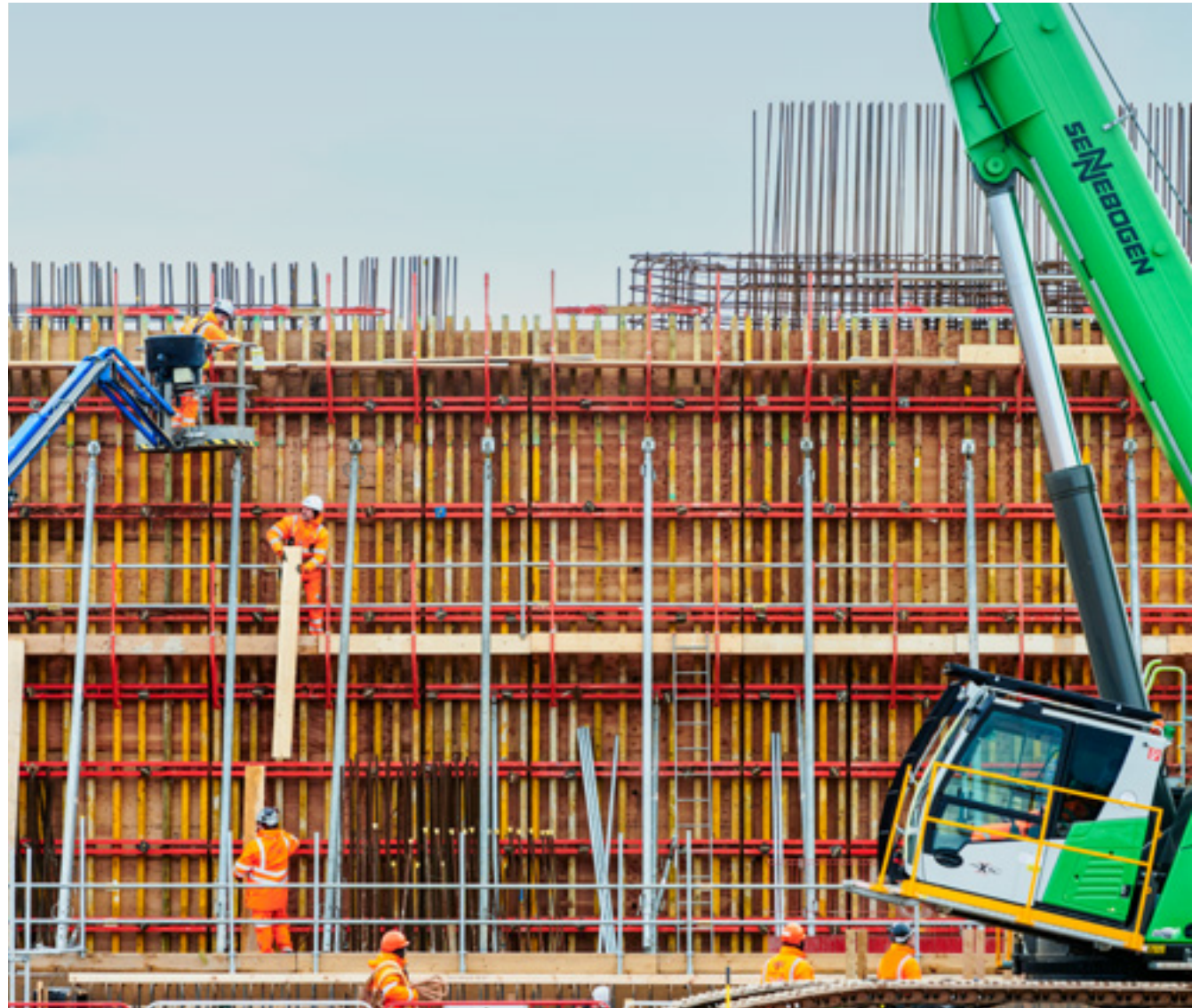
Operatives working safely at height on a Kingsbury site.
