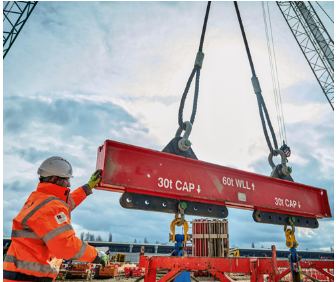
An RSJ being lifted into position at Old Oak Common station.
