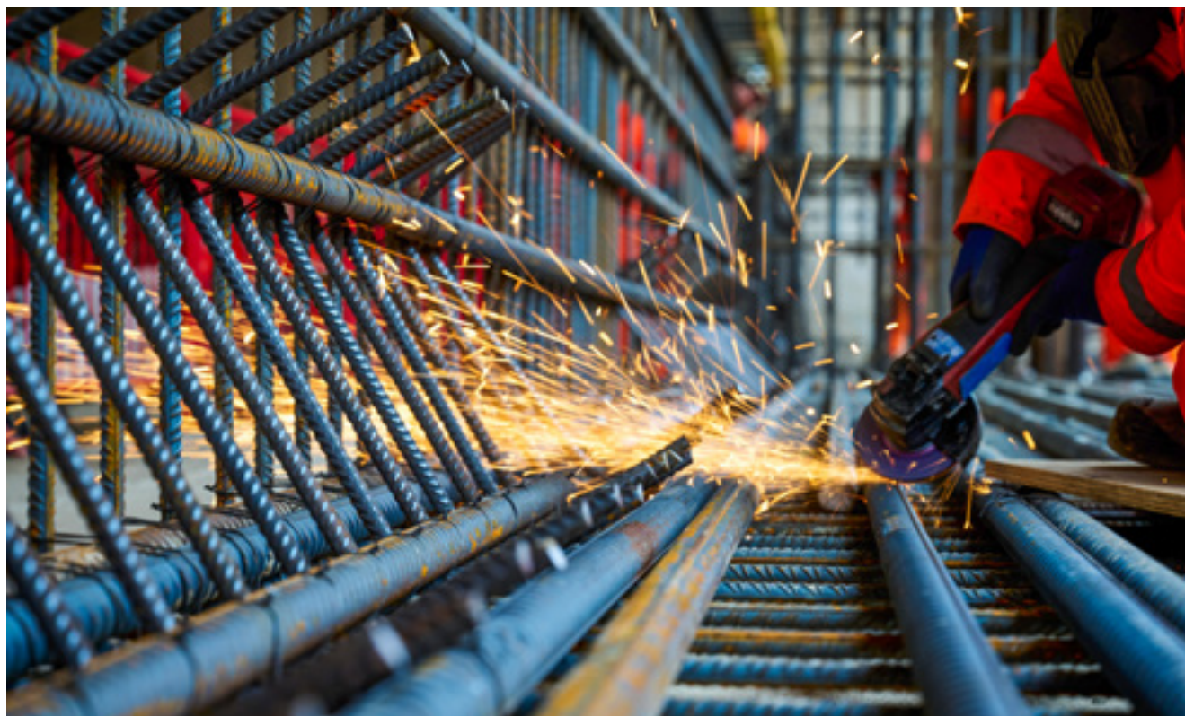
Work at Old Oak Common station.
