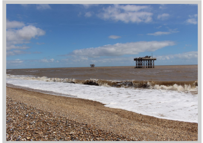
Figure 2. Cooling Water Towers
