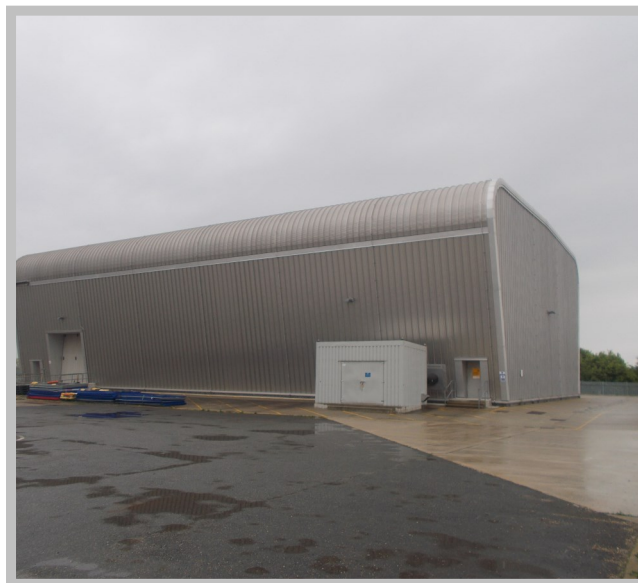
Figure 9: Bradwell Site Interim Storage Facility for ILW
