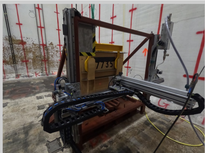
Figure 12: Skip Re-characterisation activities being carried out within the Cooling Ponds.
