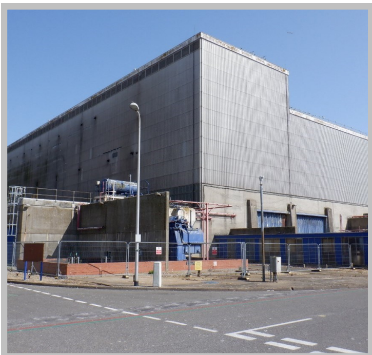
Figure 5: Turbine Hall Building
